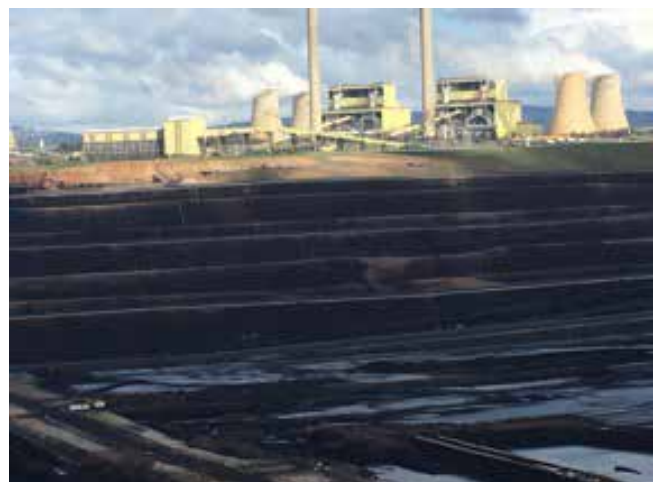
The power station with the mine in the foreground. The coal bunker is the rectangular building on the left.
