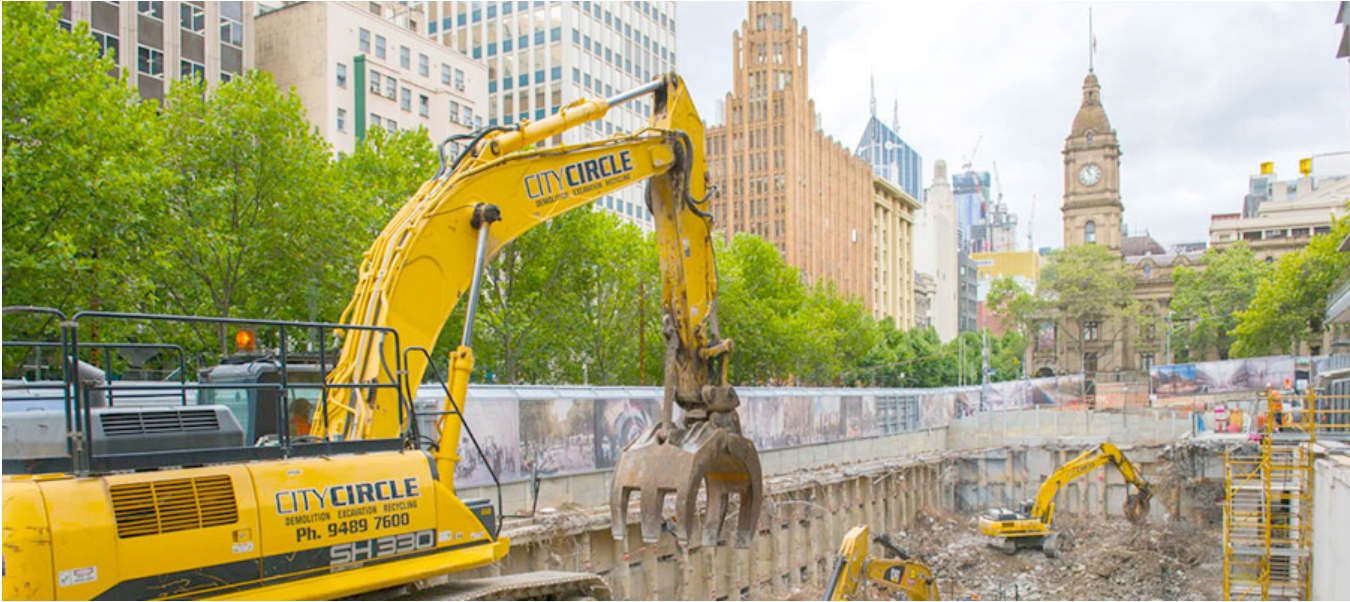
Photo: Excavation work in City Square, Melbourne CBD
