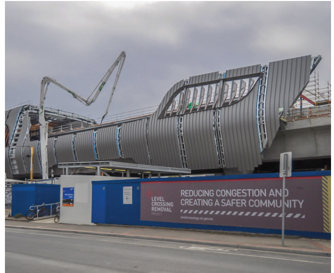
Murrumbeena Station under construction.
