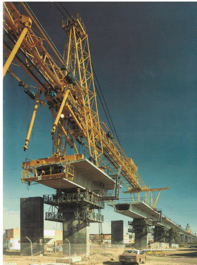
Construction of the East-bound Carriageway
