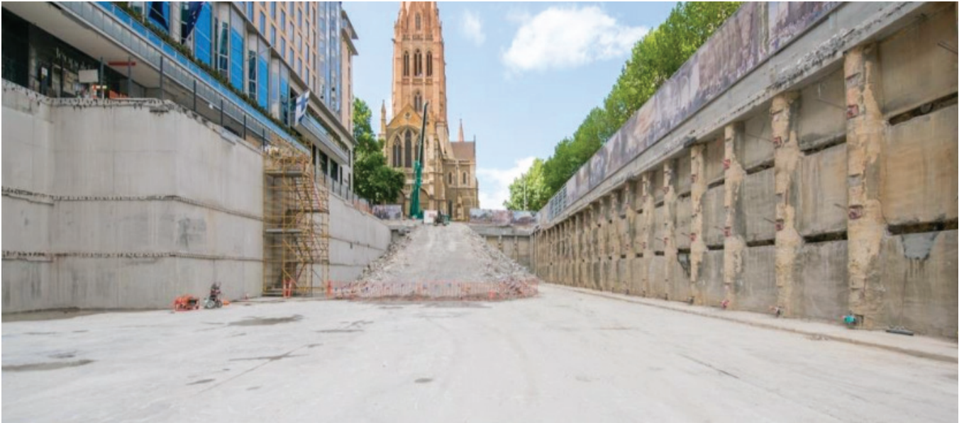
Excavation in City Square
