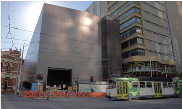
External view of the acoustic shed and construction works being carried out inside it.
