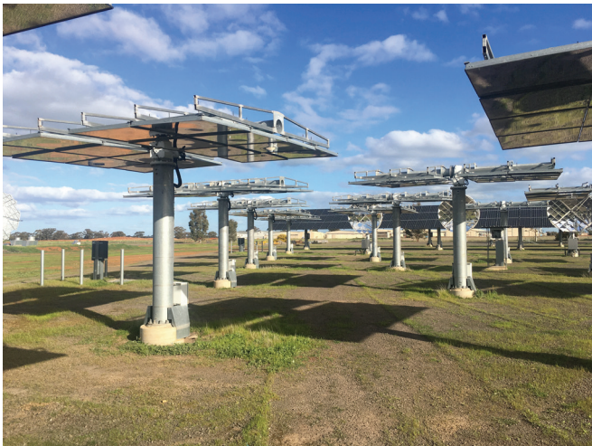
Some of the images taken at Ceramet Solar Plant.
