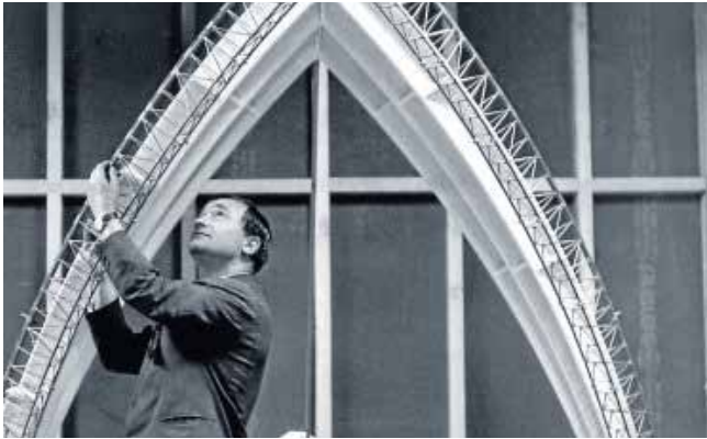
Joe Bertony at work on a model of the erection arch in 1963.
