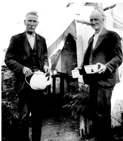
Mid 1930s – Men of the East Gippsland roads at 'home' near Bairnsdale
