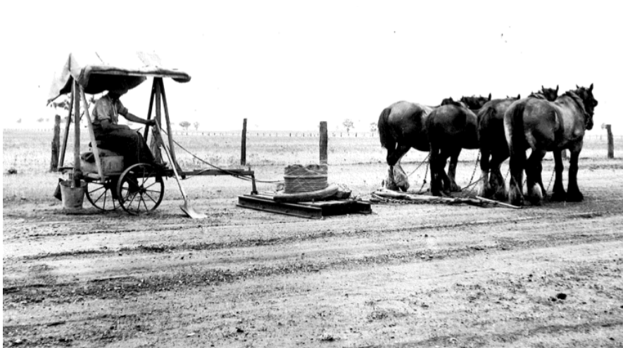
Circa 1936 – A patrolman's outfit for adverse weather conditions: dragging on the Serpentine Road in East Loddon Shire.
