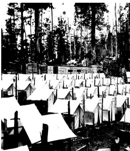
1938 – Campsite for unemployment relief road workers on the Noojee to Erica Road in Gippsland
