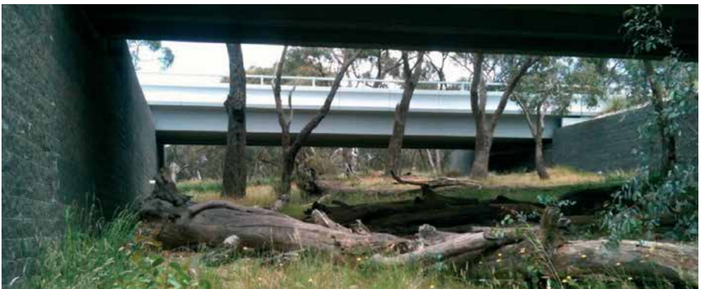
Calder freeway fauna underpass
