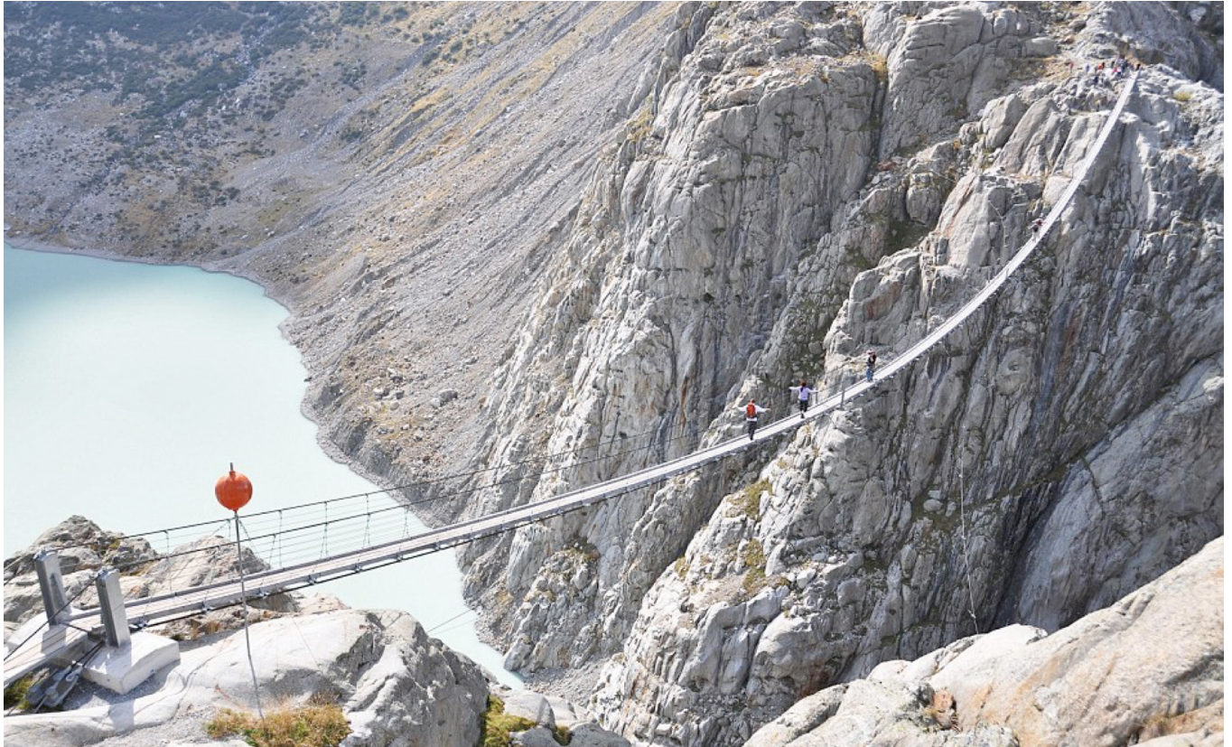
A long way to go: Trift Bridge in Switzerland is the longest pedestrian-only suspension bridge in the Alps at 557 feet in length
