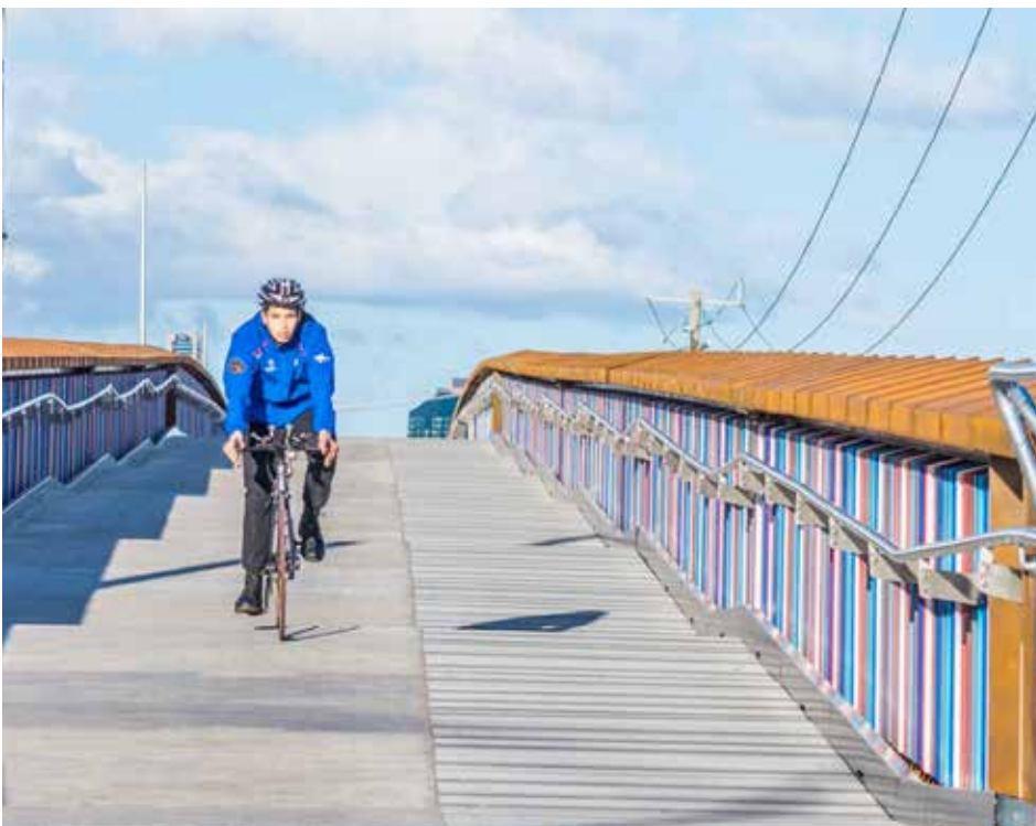
The shared facility bridge five weeks after the construction of the beams
