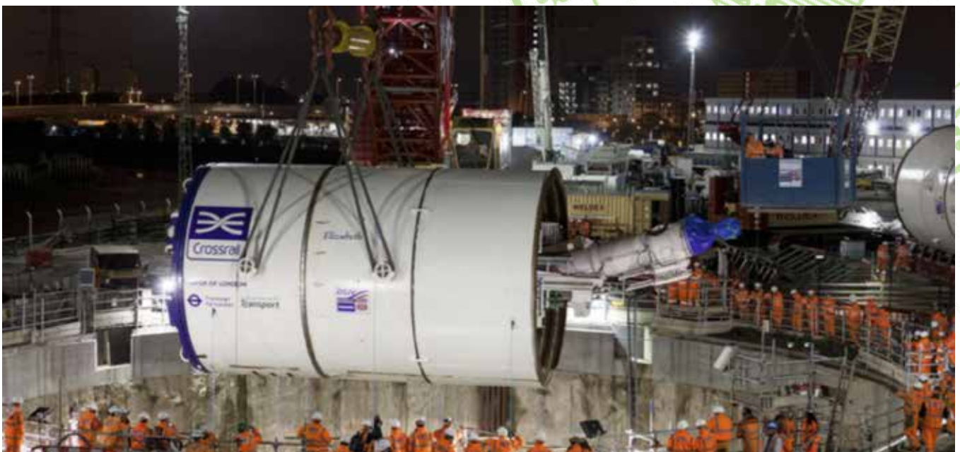
Tunnel boring machine
