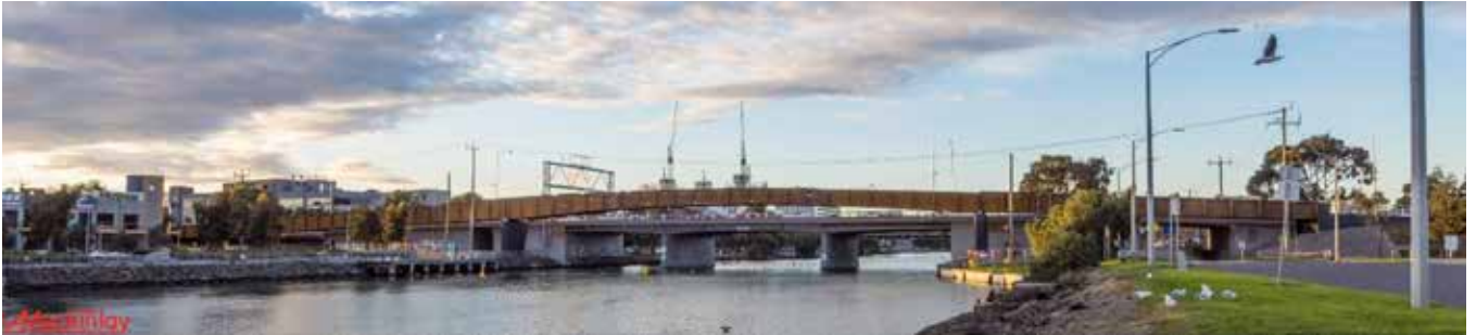
Stage 4: General view of the completed superstructure
