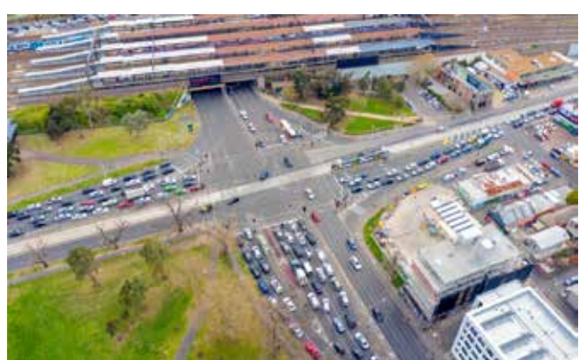
The Swan Street intersection before the CFI.
