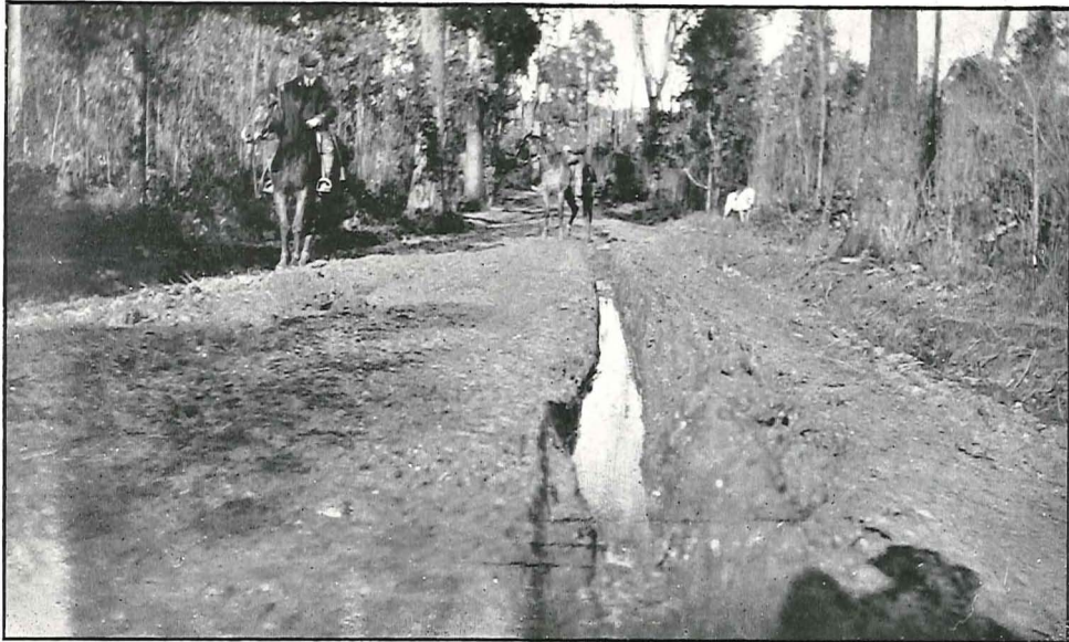
Plate 75. Showing effect of timber traffic on road in Winter.
