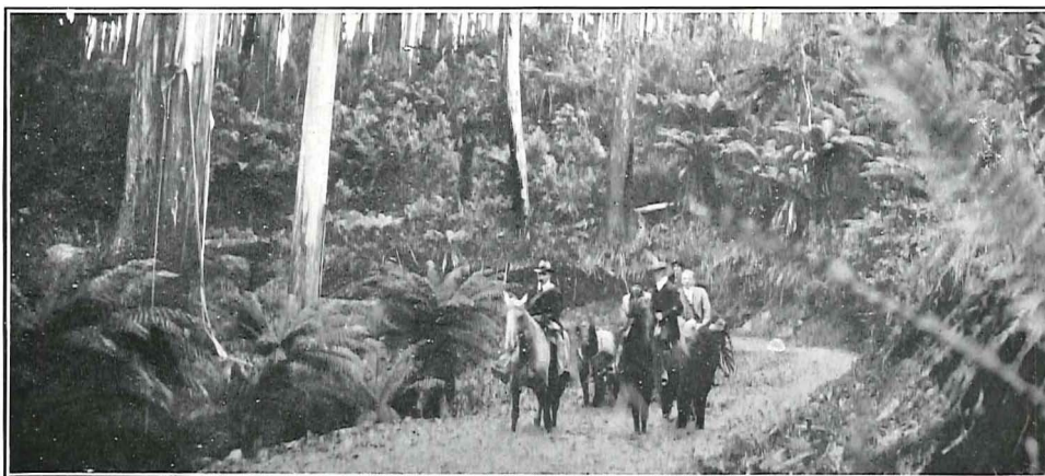
Plate 4. Showing ordinary Winter condition of a road in South Gippsland.
