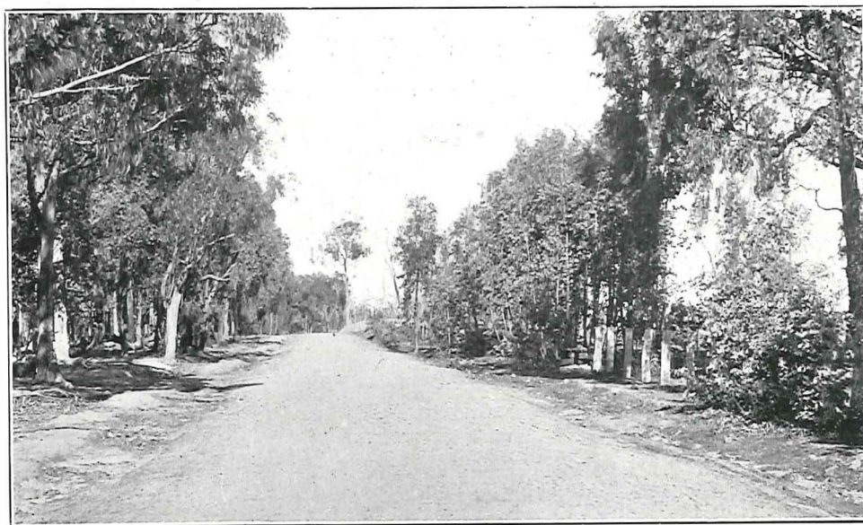
Plate 52. Showing section of the Benalla-Mansfield road, constructed of granite sand.
