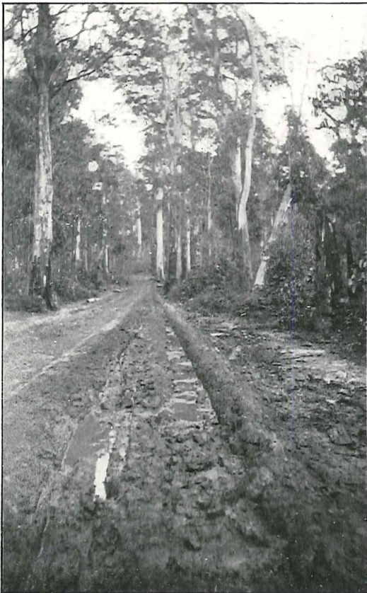
Plates 73 and 74. Showing effect of timber traffic on roads in Winter.
