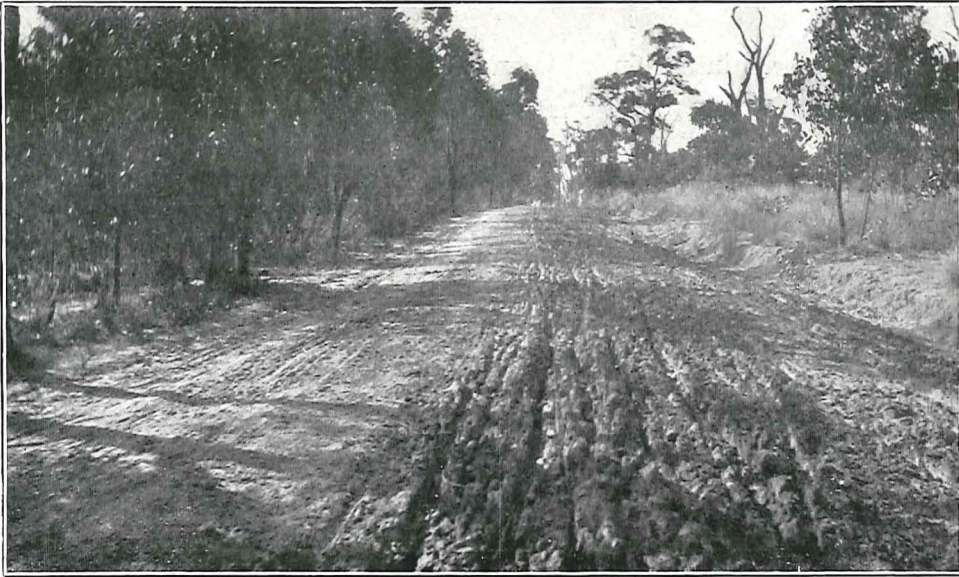
Plate 52A. Showing right and wrong use of local materials on an earth road. Left side formed of surface loam and right side with clay from gutter and bank on upper side.
