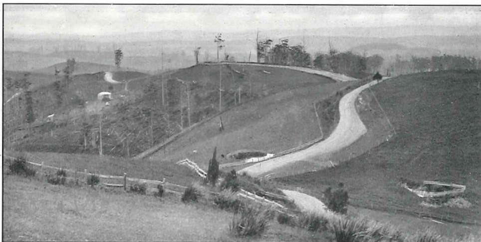
Plates 6 and 7. Showing typical location of Gippsland roads.
