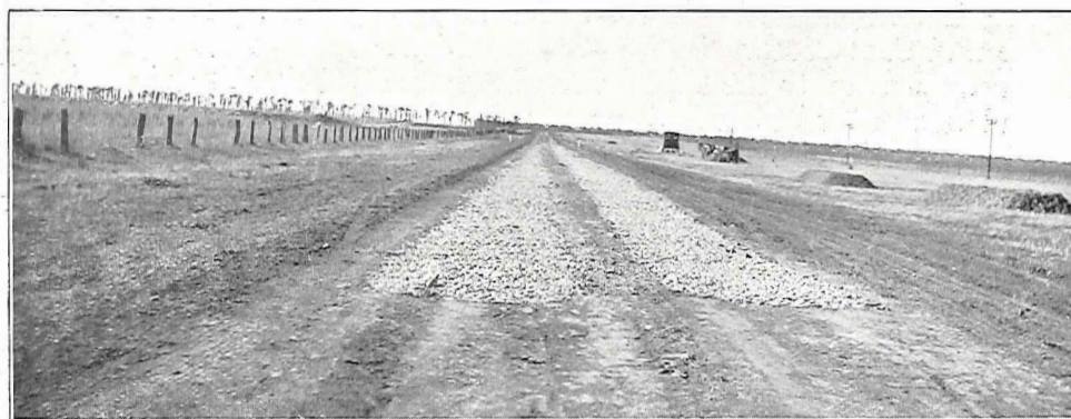
Plate 70. Showing road being repaired by the intermittent or annual system.
