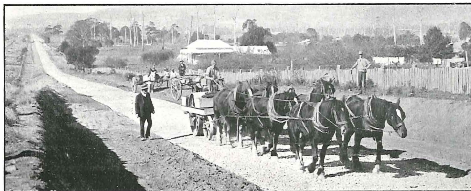
Plates 59 and 60. Showing different types of rollers now in use on country roads.
