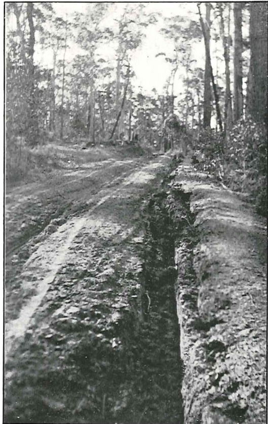
Plates 73 and 74. Showing effect of timber traffic on roads in Winter.
