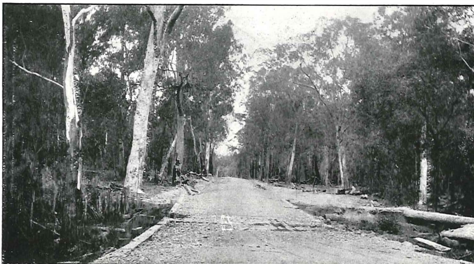
Plate 71. Good type of invert crossing on the Buchan road, constructed by the Shire Engineer of Tambo.
