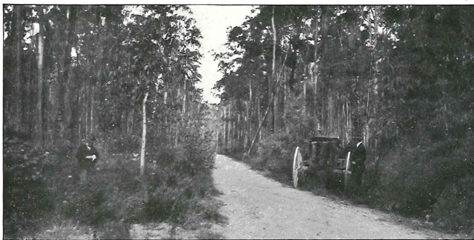
Plate 25. Showing road between Cann River and Genoa. The figure on each side shows the width originally cleared and formed six years ago.
