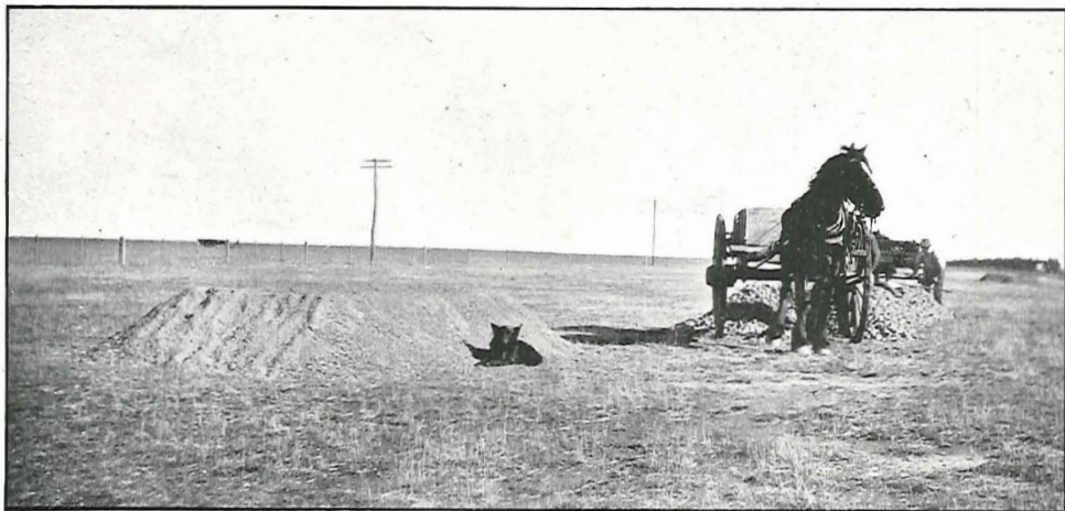
Plate 58. Showing heaps of metal and stone chippings for binder, on side of road, in the Shire of Hampden.
