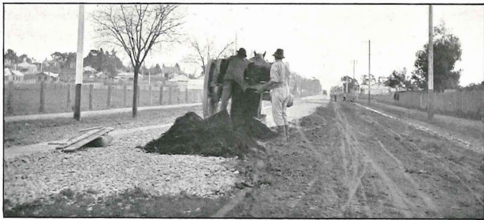
Plates 56 and 57. Showing earthy material and weeds being taken from water tables and spread on metalled roads.
