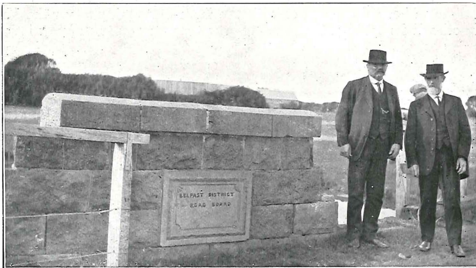
Plate 39. Showing remains of old stone culvert constructed by Belfast District Roads Board, 1856.
