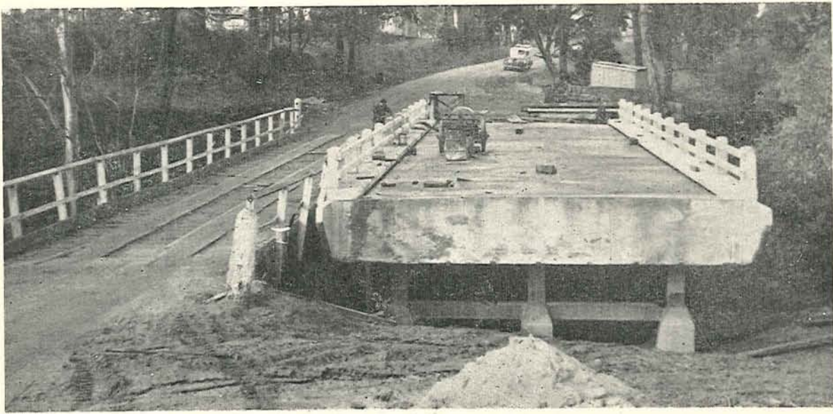
Plate No. 30.—Construction of Concrete Bridge over Bass River on the South Gippsland Highway replacing old, narrow Timber Bridge.
