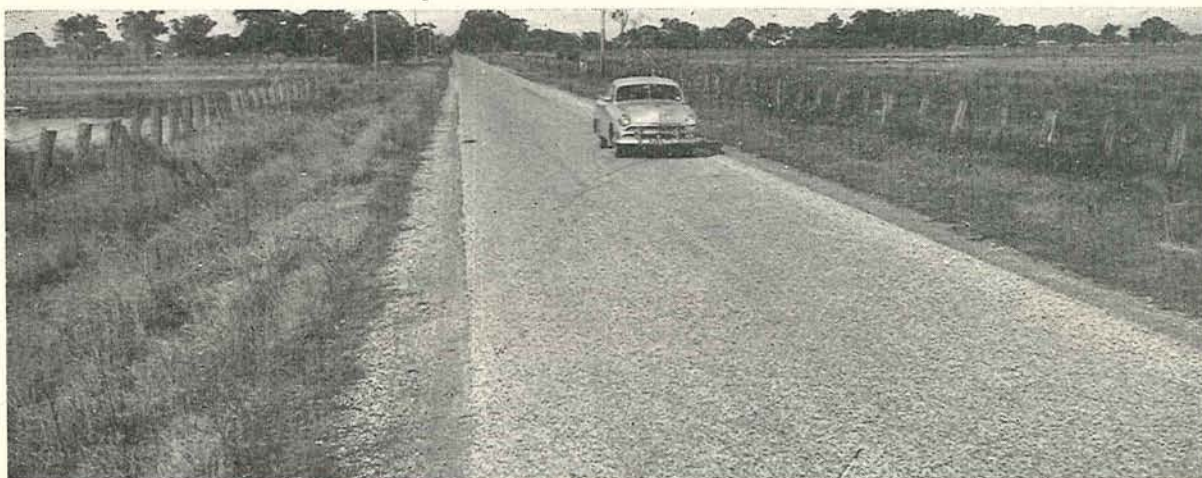
Plates Nos. 10 and 11.—Sections of the Tatura-Murchison Road. Top picture shows badly failed old sealed section two and a half miles north of Murchison. Lower picture shows a section south of Tatura saved by resealing.
