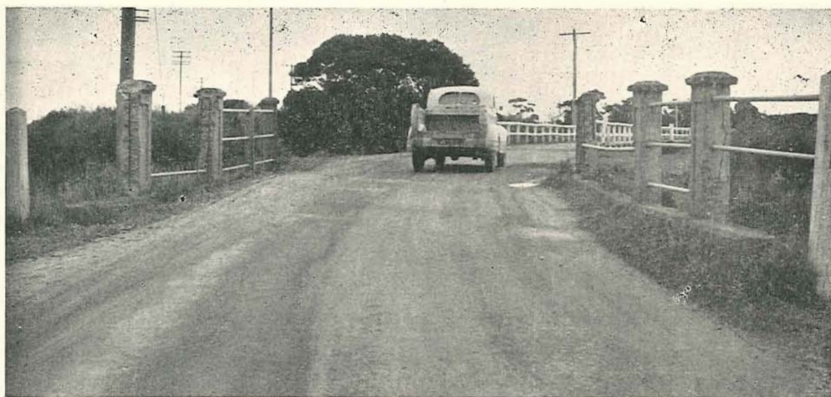
Plate No. 18.—Narrow Bridge on Curve Approaching Main Drain on the Koo-wee-rup-Pakenham Road, showing Damaged Handrail.
