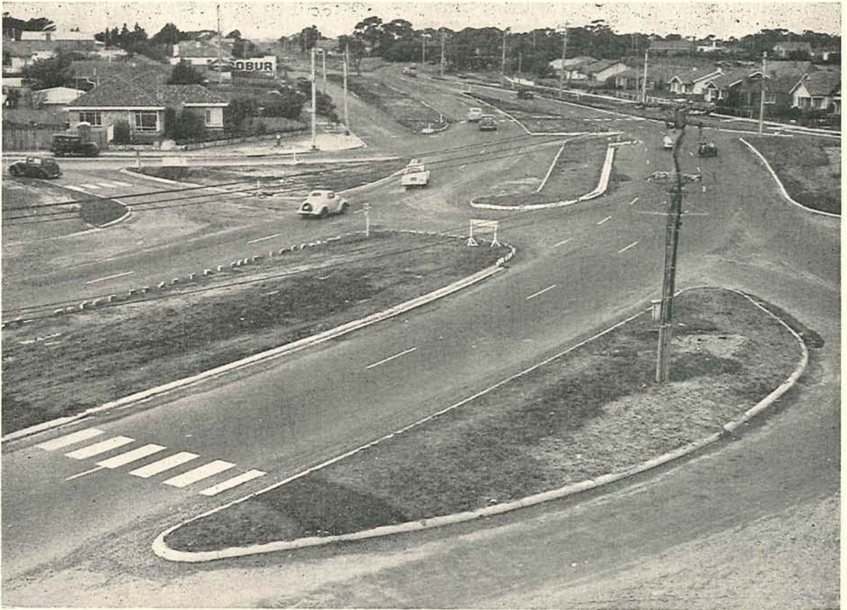
Plate No. 16.—Channelization at Corner of Nepean Highway and Warrigal Road, Mentone.
