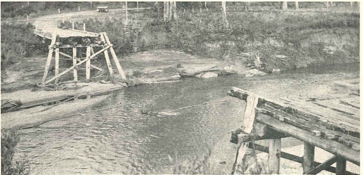
Plate No. 38.—Old Flood Damaged Bridge on Cann Valley Road at Cann River.
