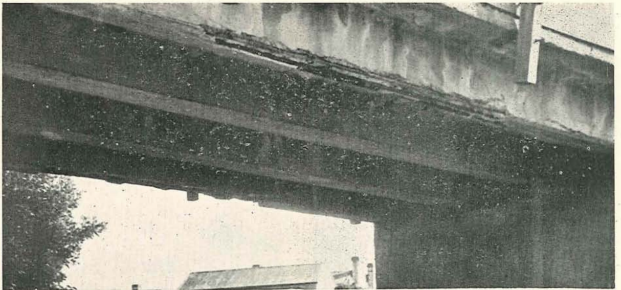
Plate No. 5.—Deterioration of Old Reinforced Concrete Bridge over Kilmore Creek on the Northern Highway.
