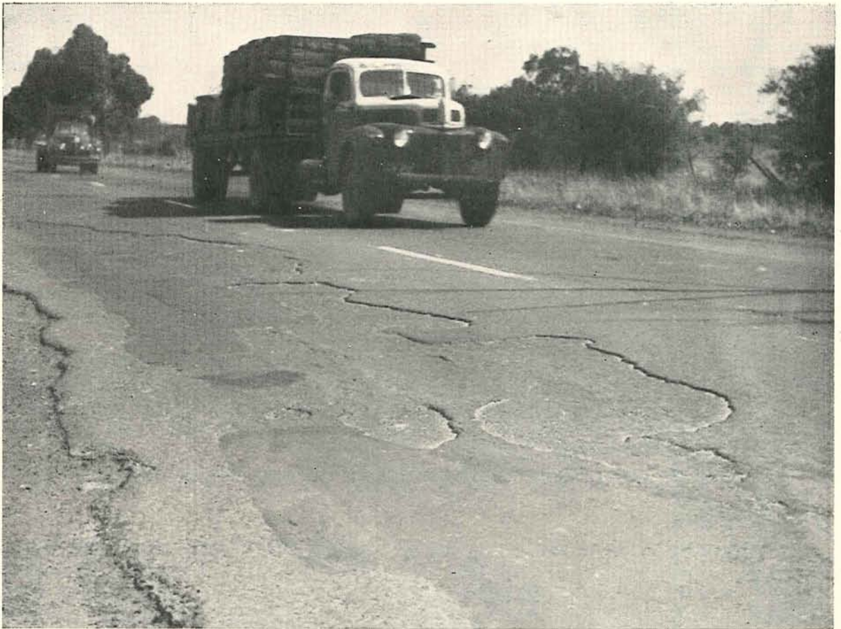
Plate No. 14.—Deteriorated Condition of Hume Highway North of Fawcner in 1951.
