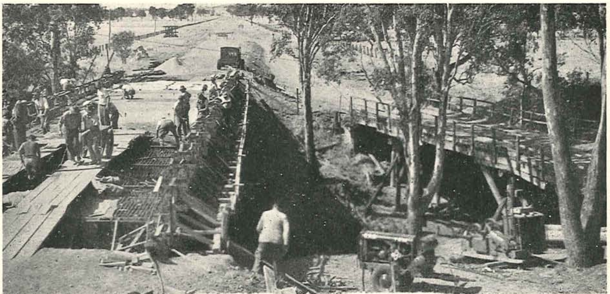
Plate No. 22.—Casting the Deck of the New Bridge.
