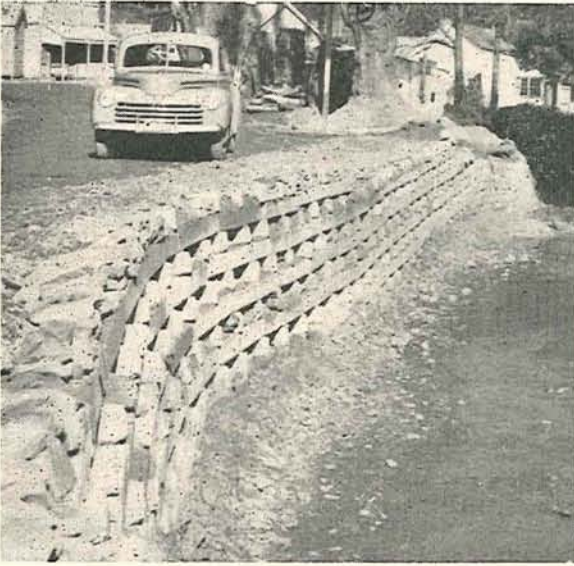
Plate No. 36.—Precast Concrete Log and Chock Type of Retaining Wall at Stringer's Creek, Walhalla.
