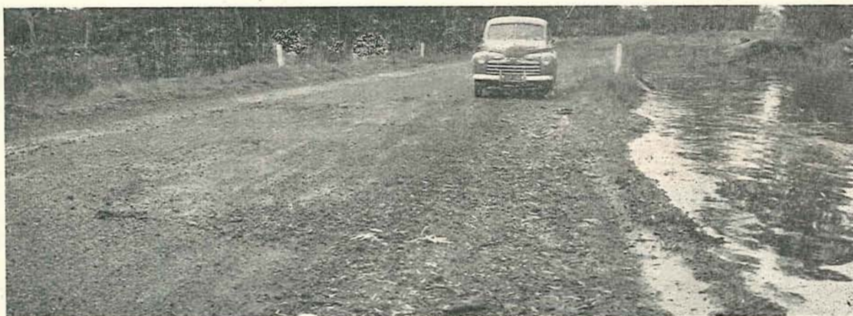
Plate No. 8.—Apsley Road seven miles north of Harrow where the high swamp level has ruined the road surface.
