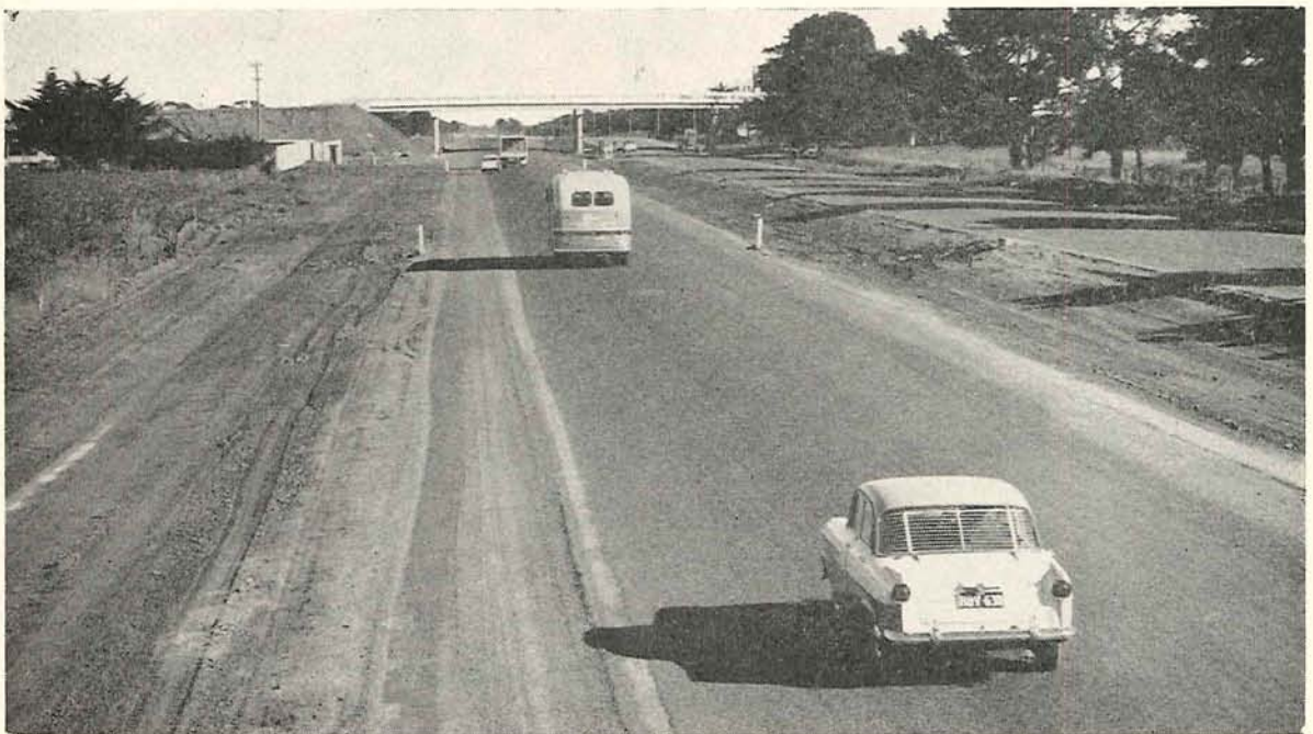
Plate 20.—Maltby By-pass. Duncan's Road Over-pass.
