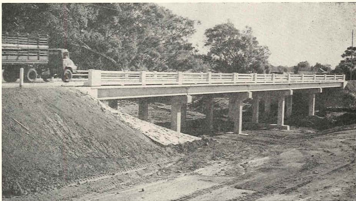
Plate 9.—Calder Highway. New bridge over Bullabul Creek.
