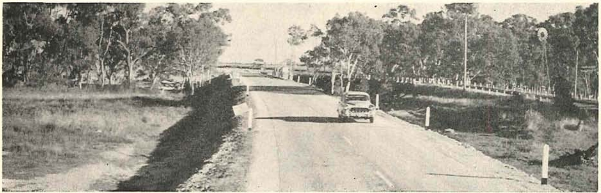
Plate 15.—Wimmera Highway. New concrete bridge over Wimmera River at Quantong.
