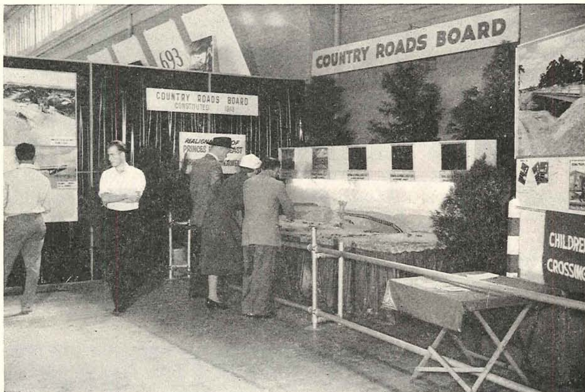
Plate 44.—Country Roads Board exhibit at Motor Show, March, 1961.
