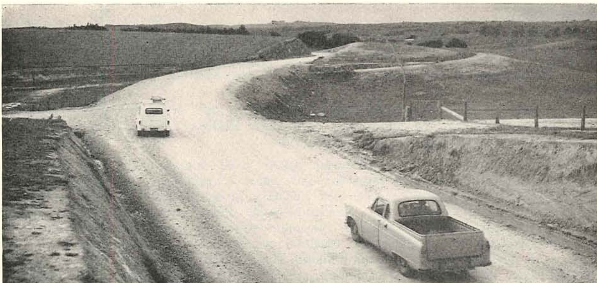
Plate 28.—South Gippsland Shire. Fish Creek—Yanakie Road. Reconstruction eliminating sharp bends south of Fish Creek.
