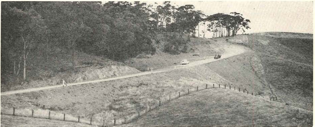
Plate 24.—After reconstruction and realignment of Wodonga-Beechworth Road approaching Indigo Creek.
