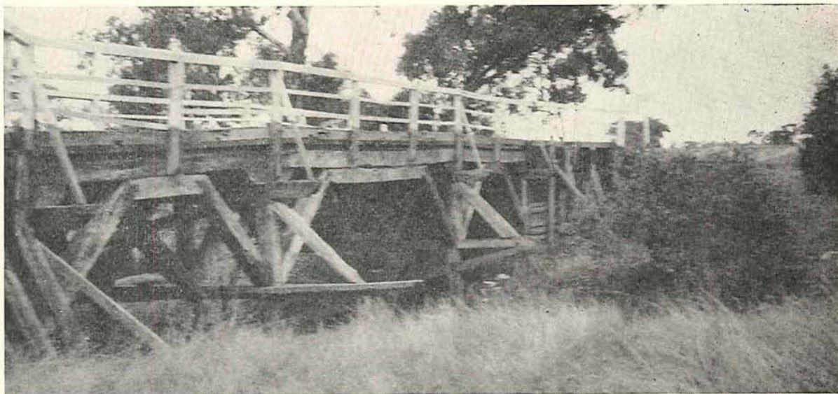
Plate 8.—Calder Highway. Old bridge over Bullabul Creek west of Bridgewater.
