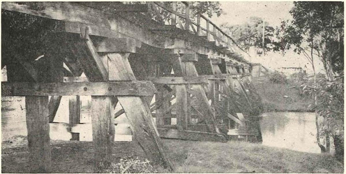
Plate 14.—Wimmera Highway. Old bridge over Wimmera River at Quantong.
