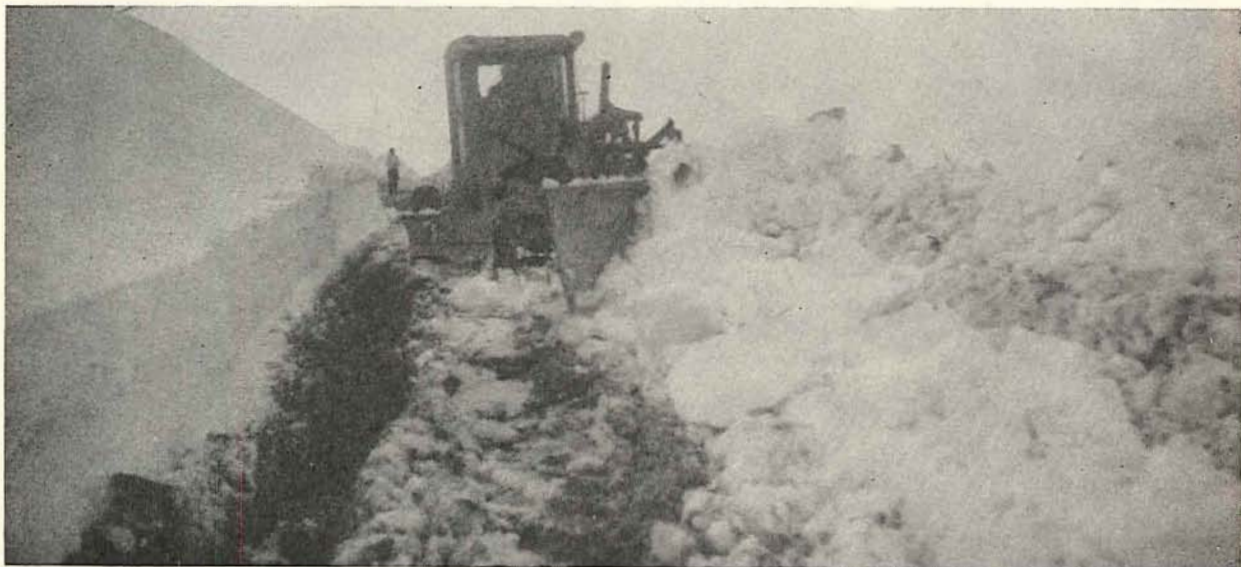
Plate 31.—Shire of Omeo. Alpine Road. Snow clearing.
