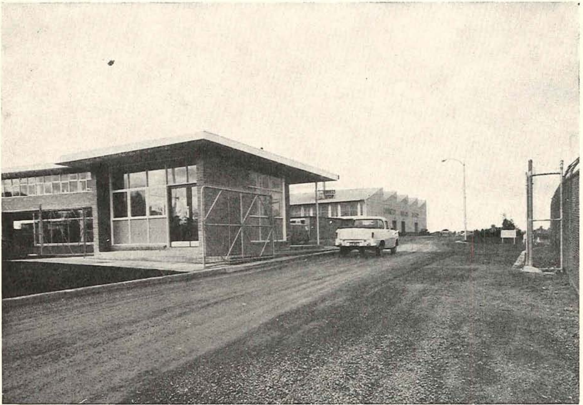
Plate 42.—Country Roads Board new workshop and office at Syndal.
