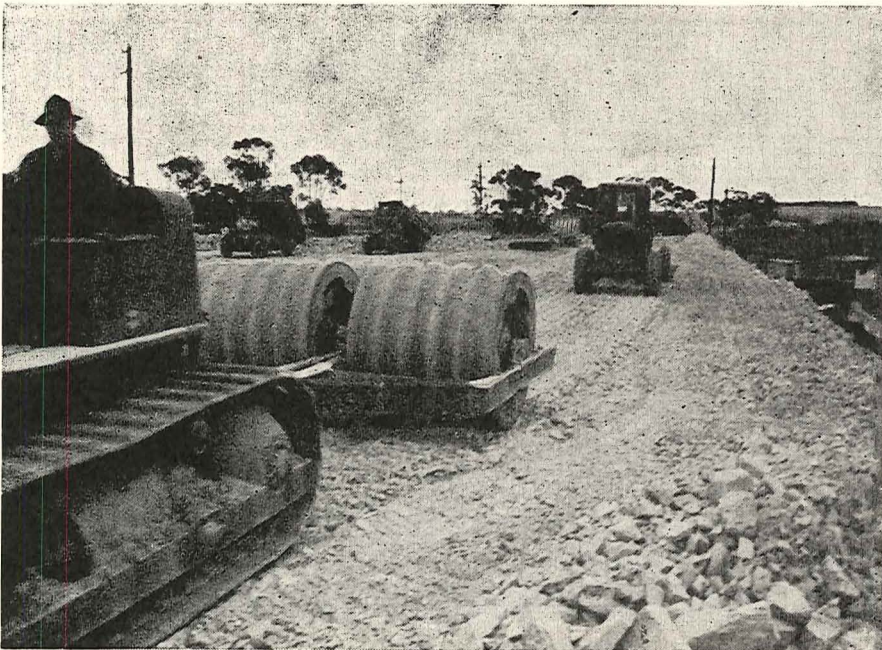
Plate 3.—Grooved roller working at Craigieburn.
