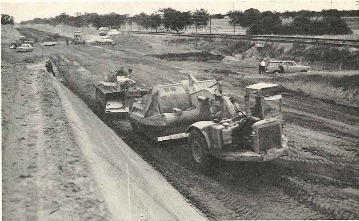
Plate 21.—Hume By-pass Road. Work in progress north of Barnawartha.
