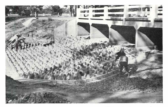
Plate 6—Placing the dissipator blocks.
