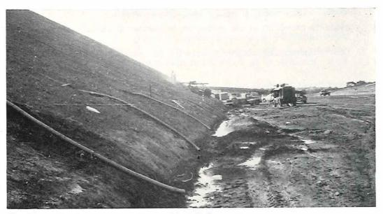
Plate 11—Drilling horizontal sub-surface drains at Mulgrave Freeway. PVC pipe is shown leading from completed drains.
