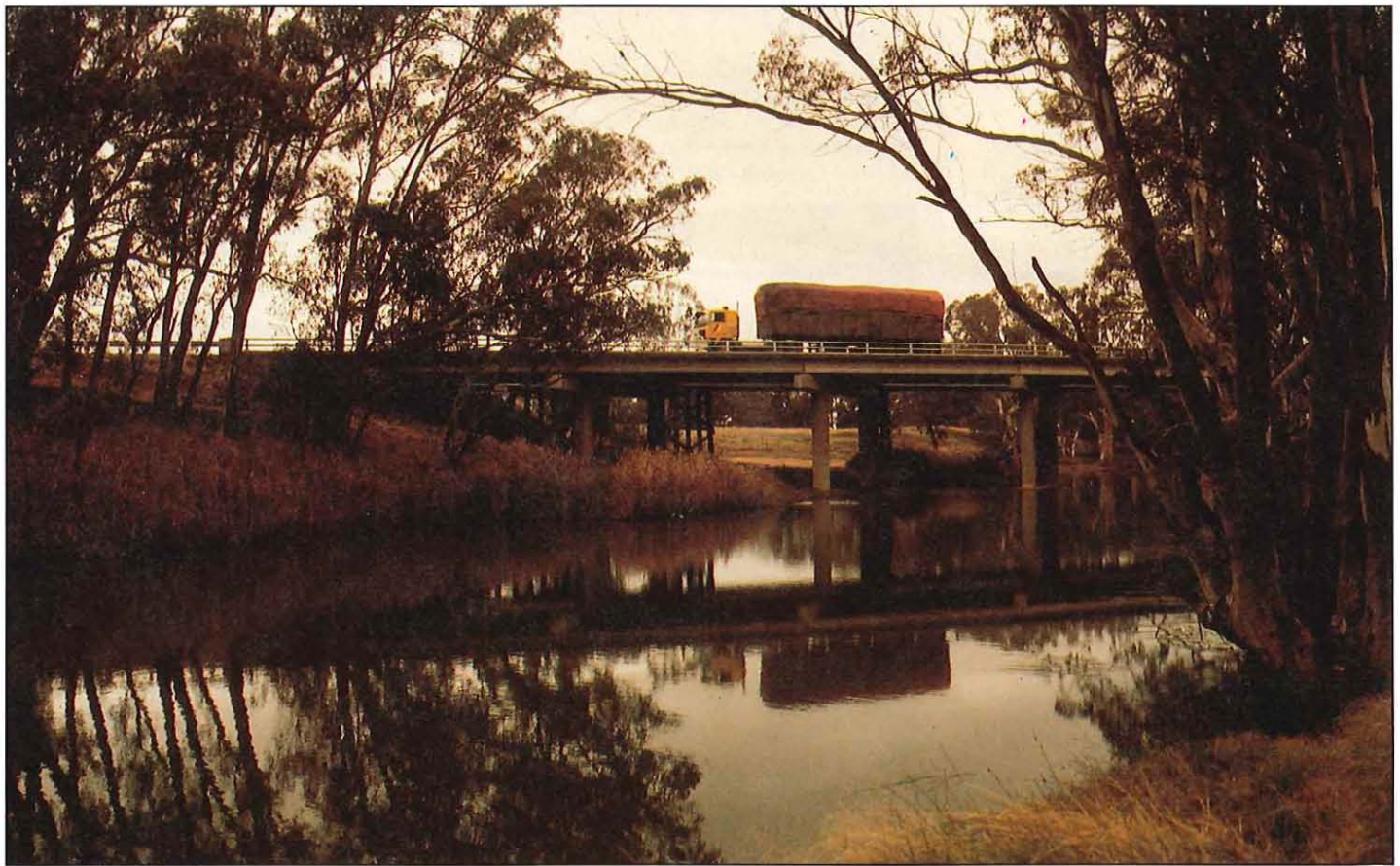
New Loddon River Bridge on the Bridgewater–Serpentine Road, south of Serpentine. The old bridge is visible in the background
