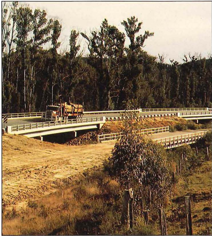
Princes Highway: new bridge over the Wingan River west of Genoa
