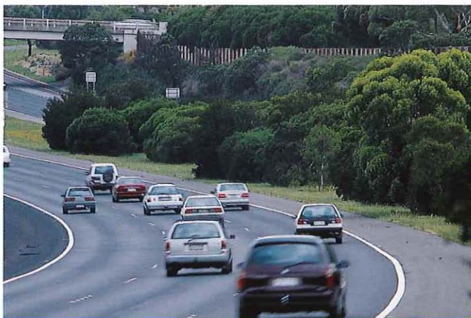
Above: In road projects, plants are selected not only for their aesthetic and environmental value, but also for their potential to minimise injury to motorists and passengers who inadvertently leave the road. Pictured are flowering Callistemon shrubs on the Monash Freeway in Mulgrave.
