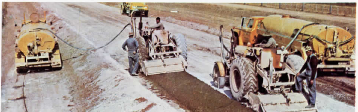
Reconstruction of the Northern Highway north of Rochester
