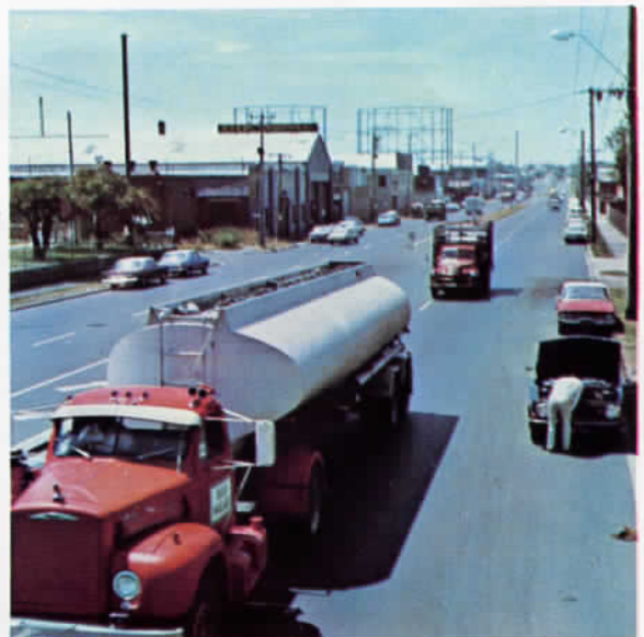
Dual carriageways in Hyde Street, Footscray
