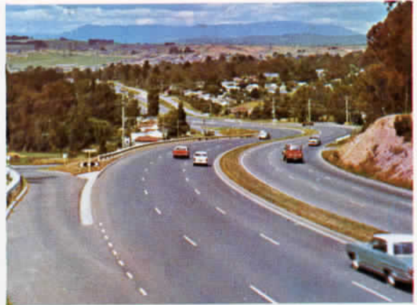
The Maroondah Highway, North Croydon
