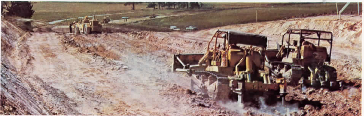
Reconstruction of the Midland Highway near Mt. Franklin
