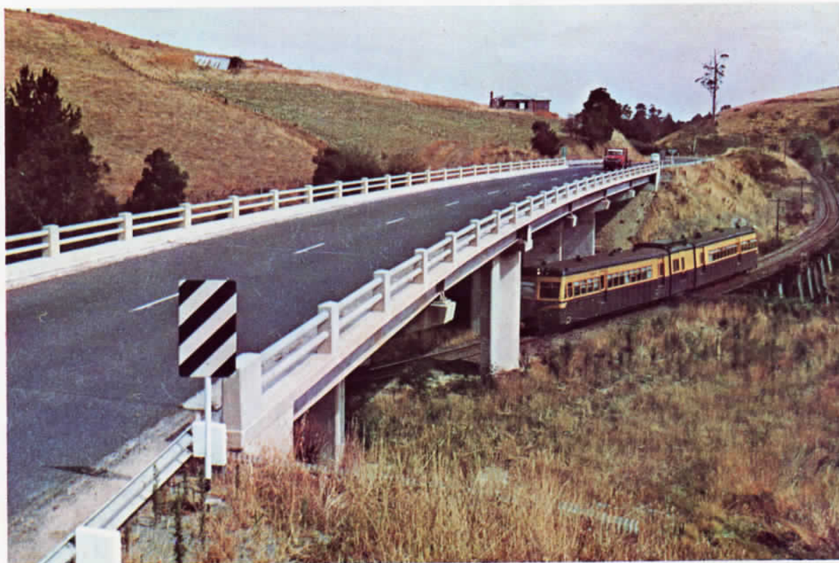
Railway level crossing eliminated on the Fish Creek - Foster Road at Hoddle
