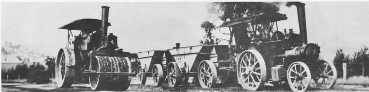
Plant working on the Maroondah Highway at Coldstream in 1928
