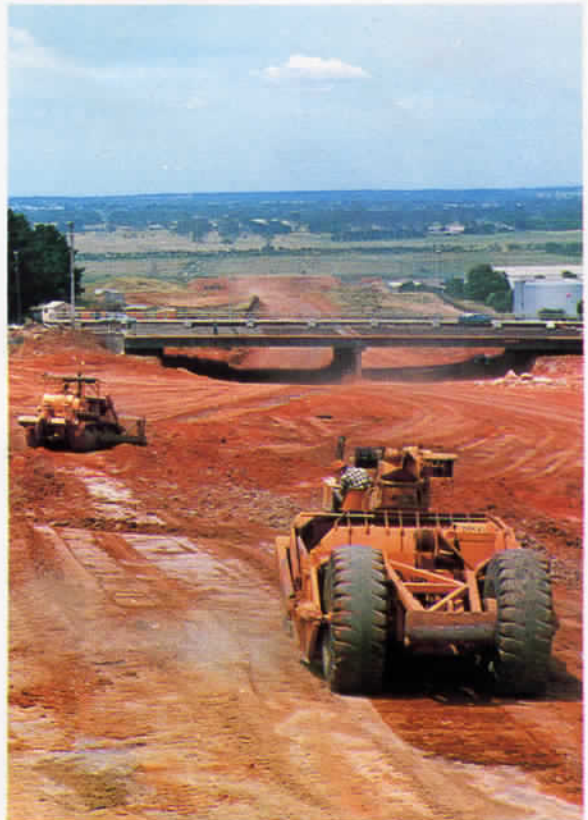
The Eumemmerring Freeway under construction
