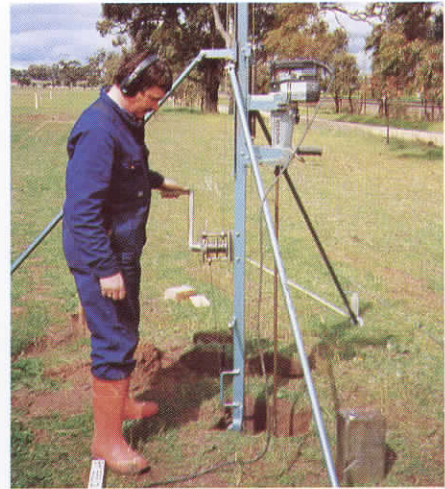
The installation of survey marks in expansive soils.
