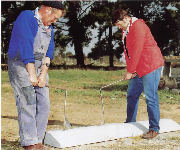
1,2,3 LIFT! It's much easier with this spike kerbing lifting device.
