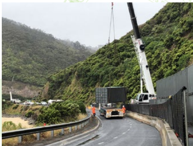
Installing the container wall barrier.
