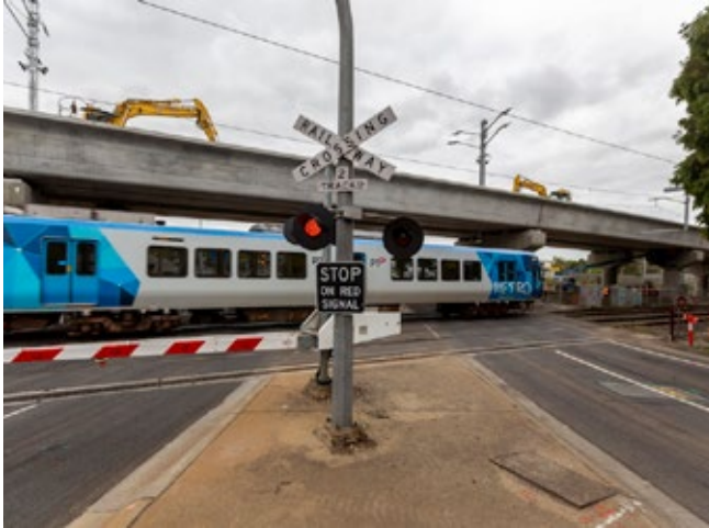
Construction of the railway overpass at the level crossing.
