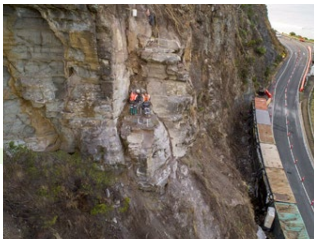
Workers dislodging rocks with the container wall barrier below.
