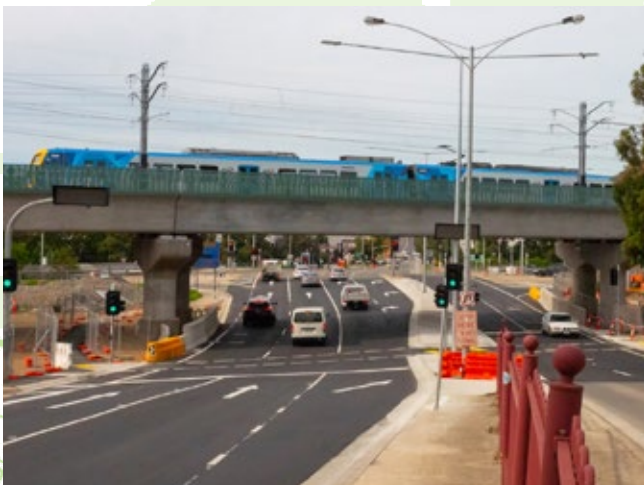
Completion of the grade separation after opening to traffic
