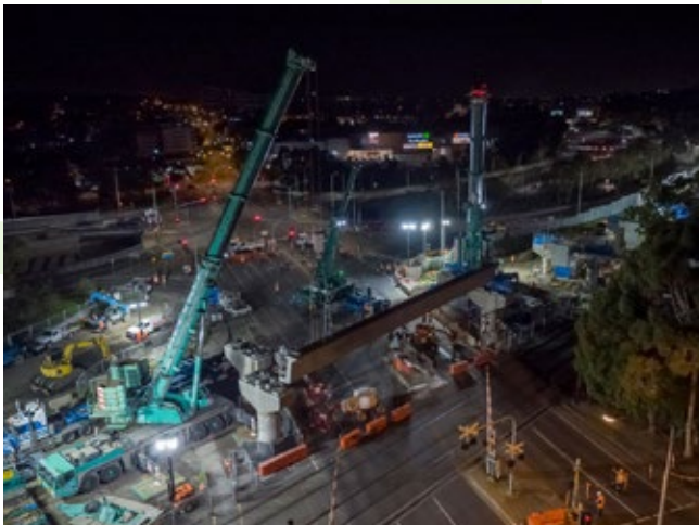
Lifting the bridge beams into place.
