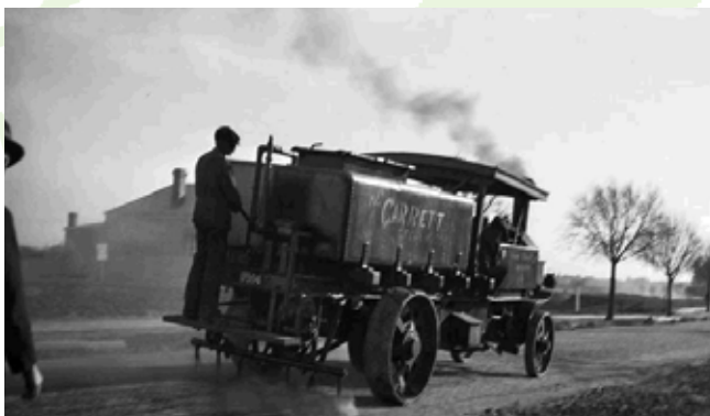
The first 900 gallon tar sprayer on the Main Healesville Road – 1914
