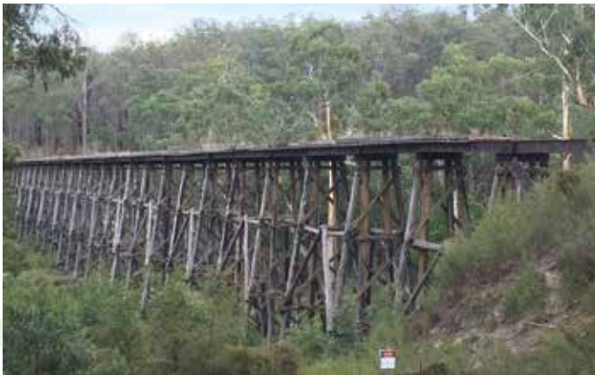
The Stony Creek trestle bridge at Nowa Nowa.
