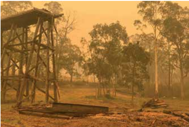
Wairewa's historic timber railway bridge was destroyed in the fire.
