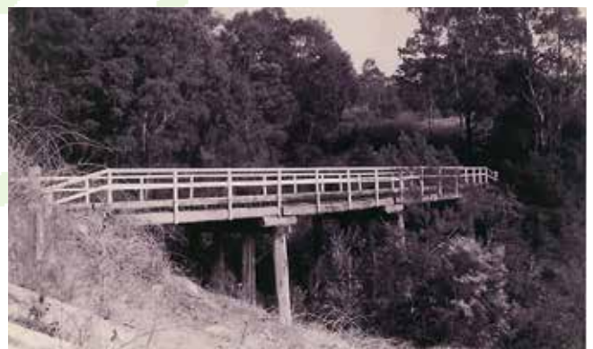
Bete Bolong Creek bridge was totally destroyed.
