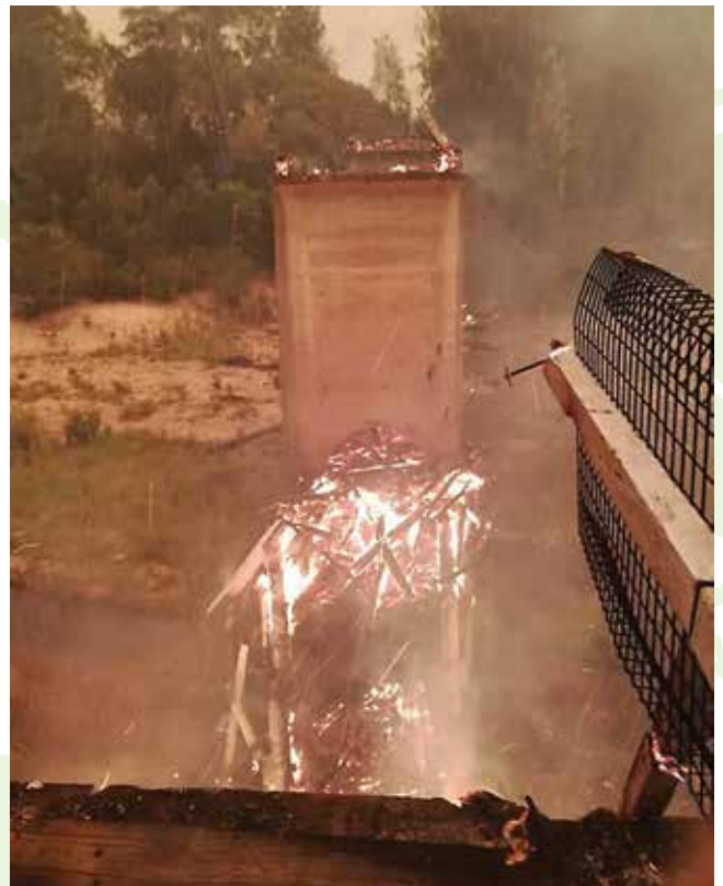
After the trusses ignited the bridge collapsed into the Genoa River.
