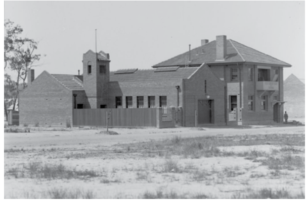
Yallourn fire station, 1920s
