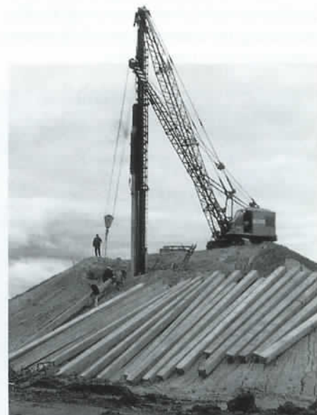
Driving the piles on Midland Highway bridge.
