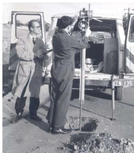
Static cone penetrometer
