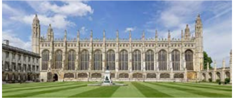
External view of the chapel.
