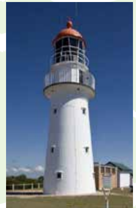
Bustard Head Lighthouse, made using prefabricated segments of cast iron bolted together.
