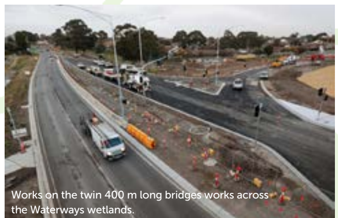
Asphalting works at the Centre Dandenong Road entry ramp – June 2021.
