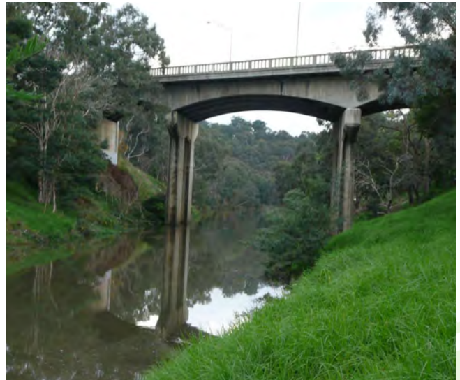
Johnston Street Bridge.
