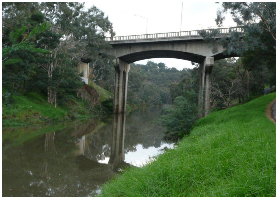
Johnston Street Bridge.
