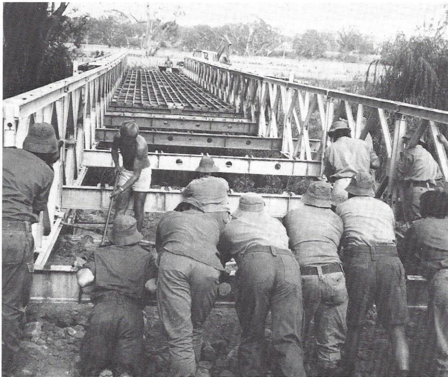
● Delaunching the bridge by manually pushing it across the stream.
