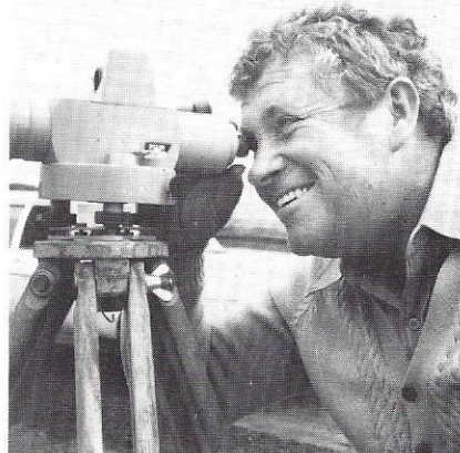
● Roadworks Overseer Frank Dwyer checks levels on the pavement. Frank has worked in Ballarat Division for 29 years.
