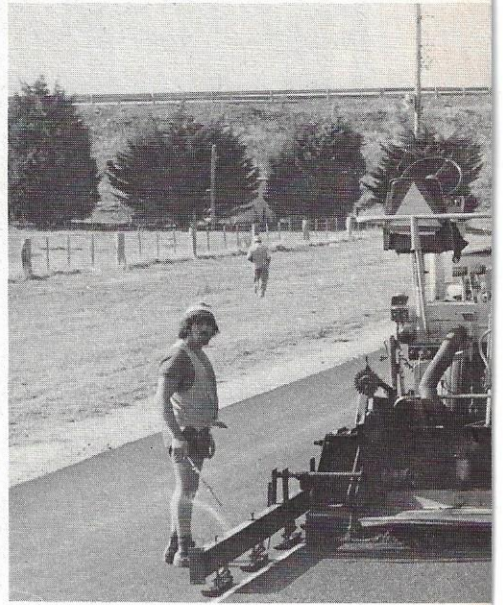
● Asphalt pavers resurface the full width
