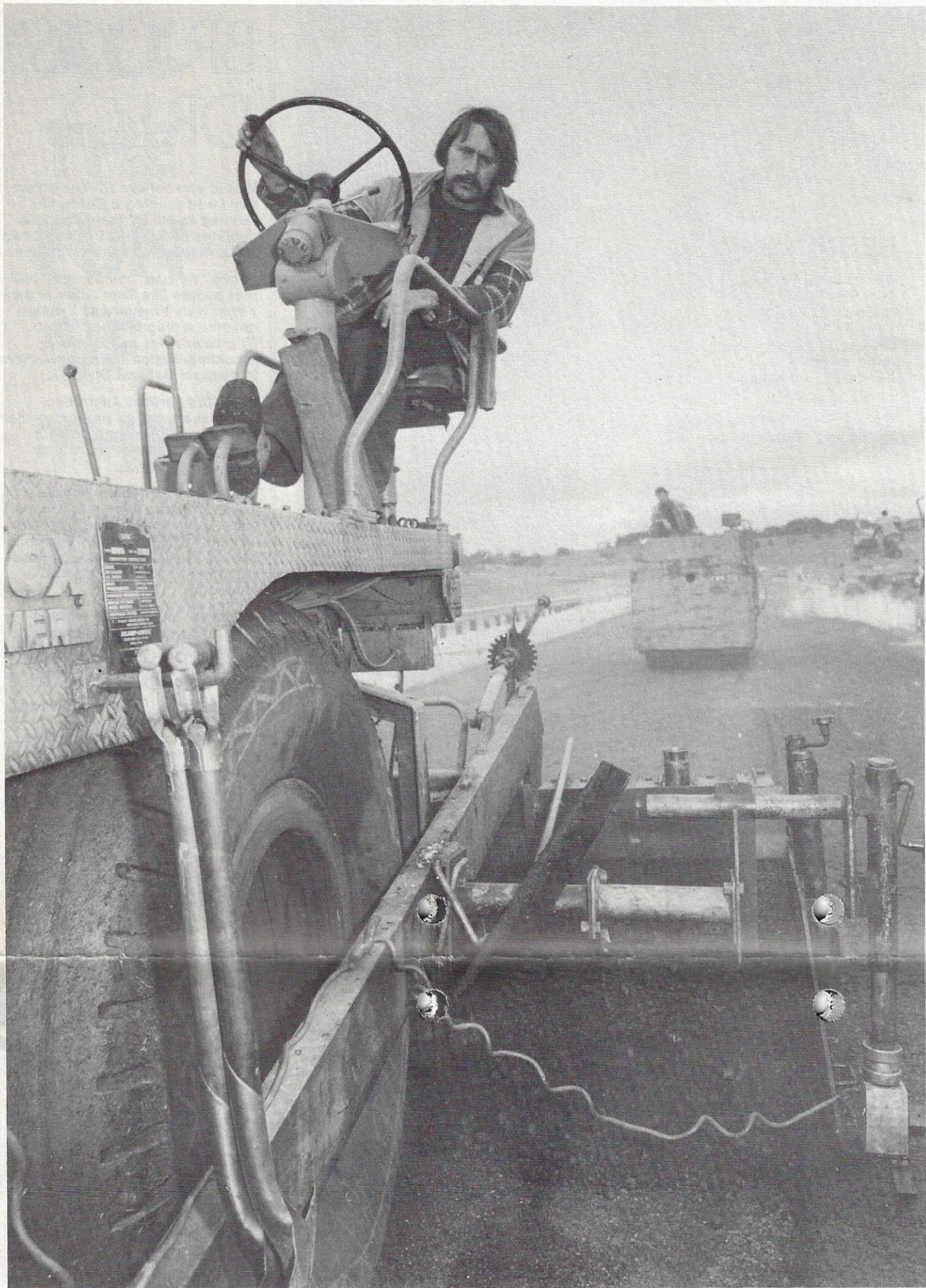
● Asphalt paving in progress on the Hume Freeway. Behind the paver is a roller.
