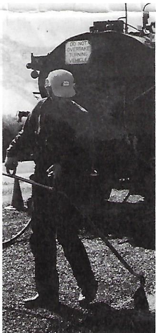
Some of Paul's 'closely knit spray crew' at work on Stud Road, Rowville. Above Left: Sprayer driver, Les Doak, uses the hand lance on a section of road. Above Right: Traffic Controller, Merv Ross, on the job. Below: Sprayer Operator, Ernie Hade, adjusts the controls on the sprayer in preparation for a spray run.
