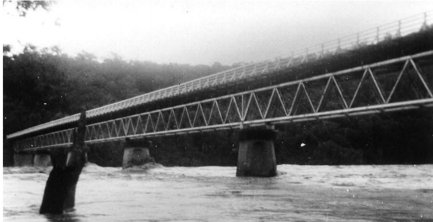
McKillops Bridge surviving a subsequent flood. VicRoads.
