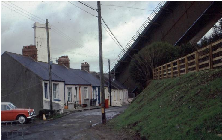
Steep approach to Milford Haven bridge in Wales in early 1970. Actually, the bridge fell conveniently into a street between two rows of houses. Photo by author.
