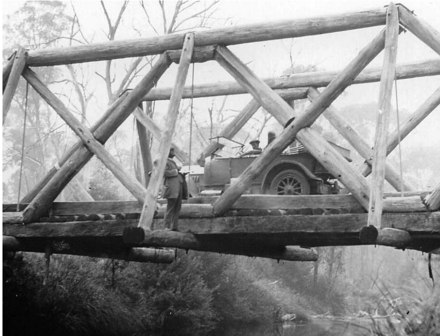
Victorian bridge designer puts reputation on the log. VicRoads
