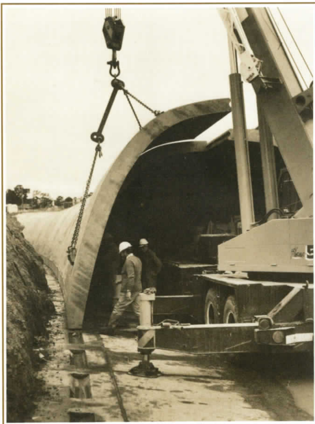
Relocating Koonung Creek in an underground conduit on the Arterial Road Extension of the Eastern Freeway, 1982
