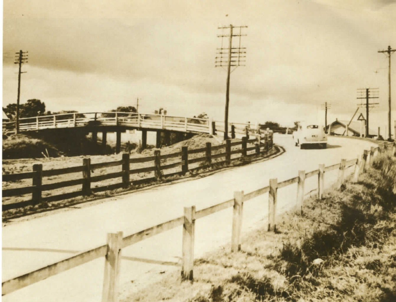
Princes Highway bridge over railway crossing at Moe, 1947
