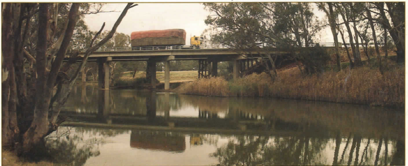
Loddon River bridge on the Bridgewater - Serpentine Road
