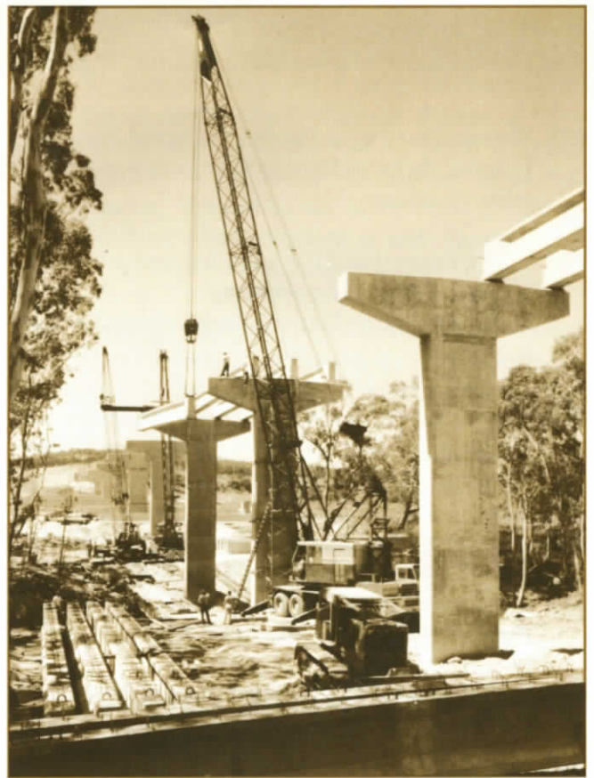
Glenelg River bridge on Princes Highway, Dartmoor, 1968
