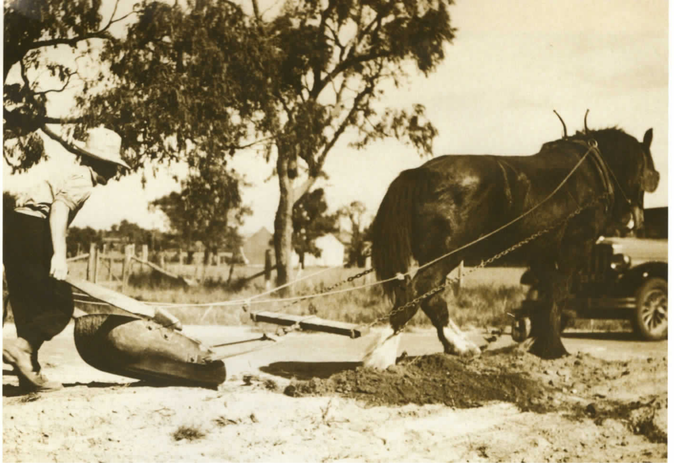
Horse drawn scoop on South Gippsland Highway west of Loch, 1948
