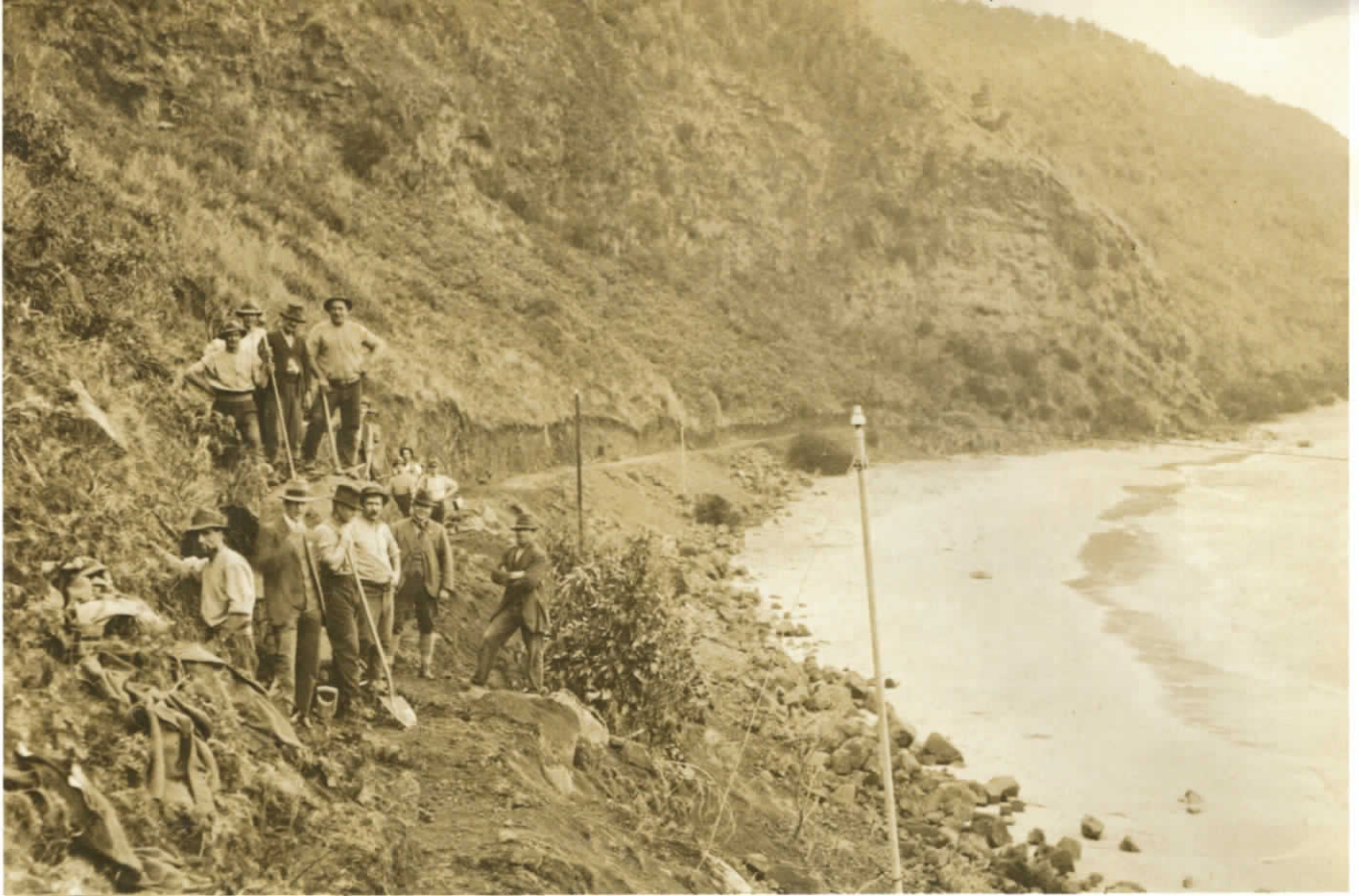
Early construction on the Great Ocean Road near Lorne
