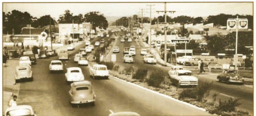
Duplication of the Maroondah Highway at Blackburn, 1961
