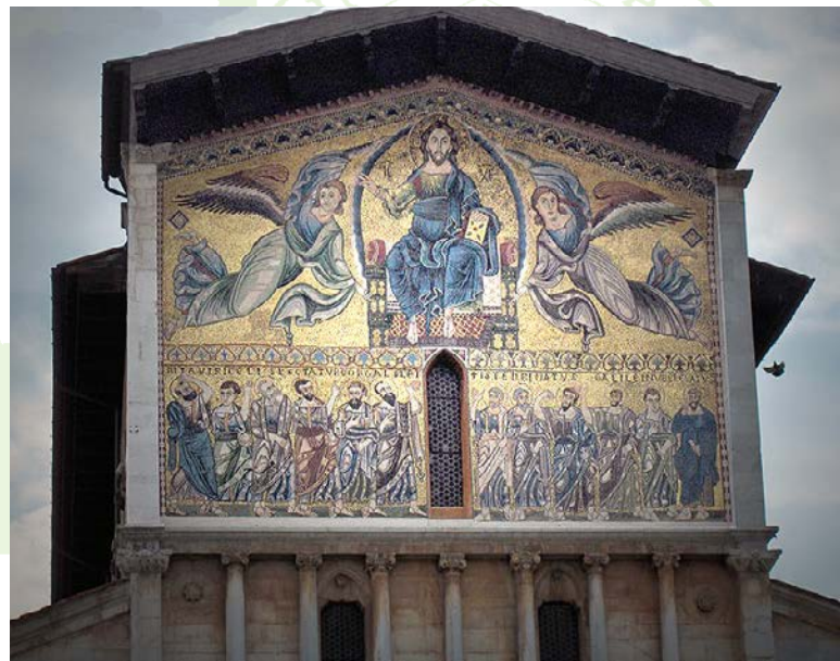
The renovated façade of San Frediano.
