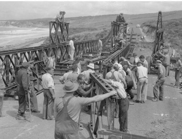
Assembling the Bailey bridge. Alec is in the white shirt, third from the left.
