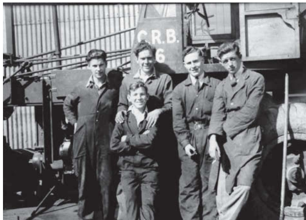
CRB staff working on the airfield at Avalon.
