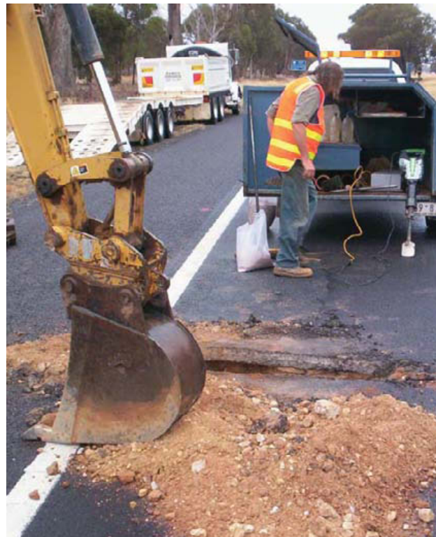
Pavement testing in progress.
