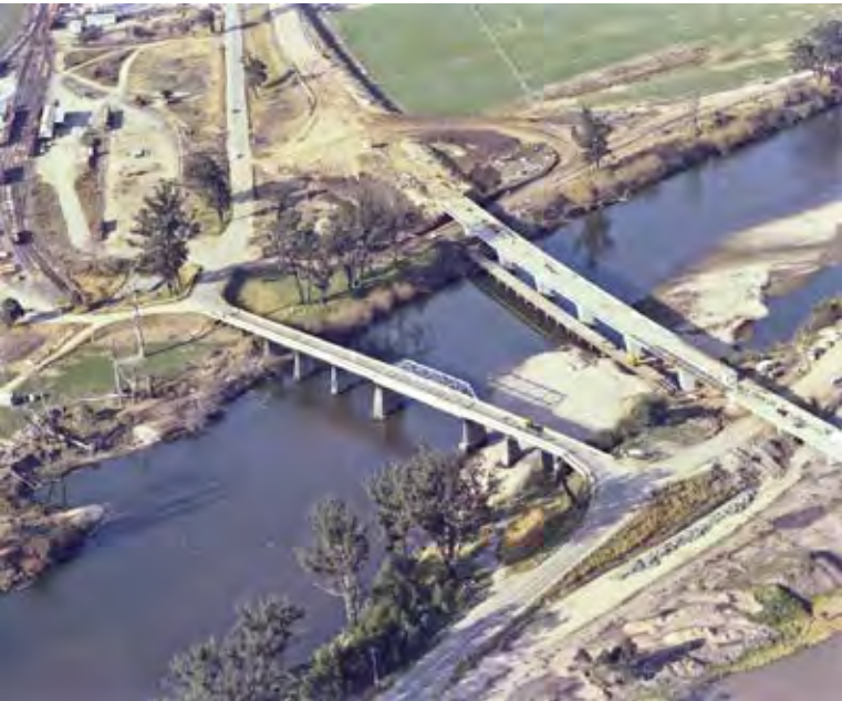
Construction of the bridge across the Snowy River – circa 1976. The old bridge is in the foreground.
