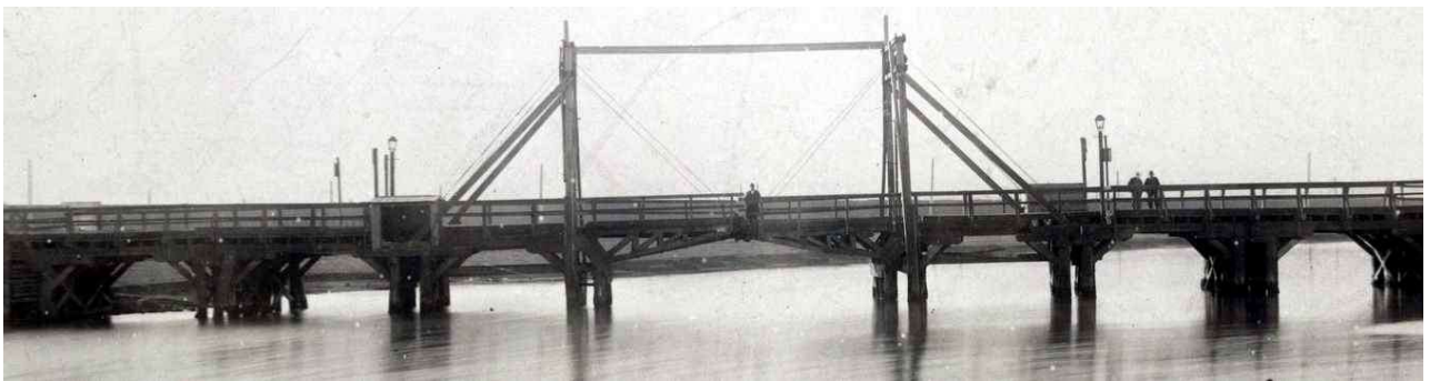
Figure 4.1c Saltwater Bridge with lift mechanism for centre span.
