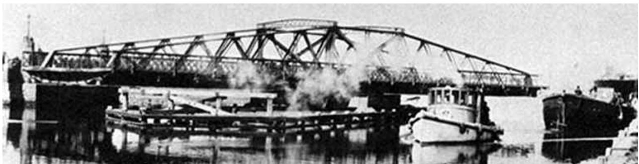
Figures 4.1e & f. The latter shows the Swing Bridge passing river traffic.
