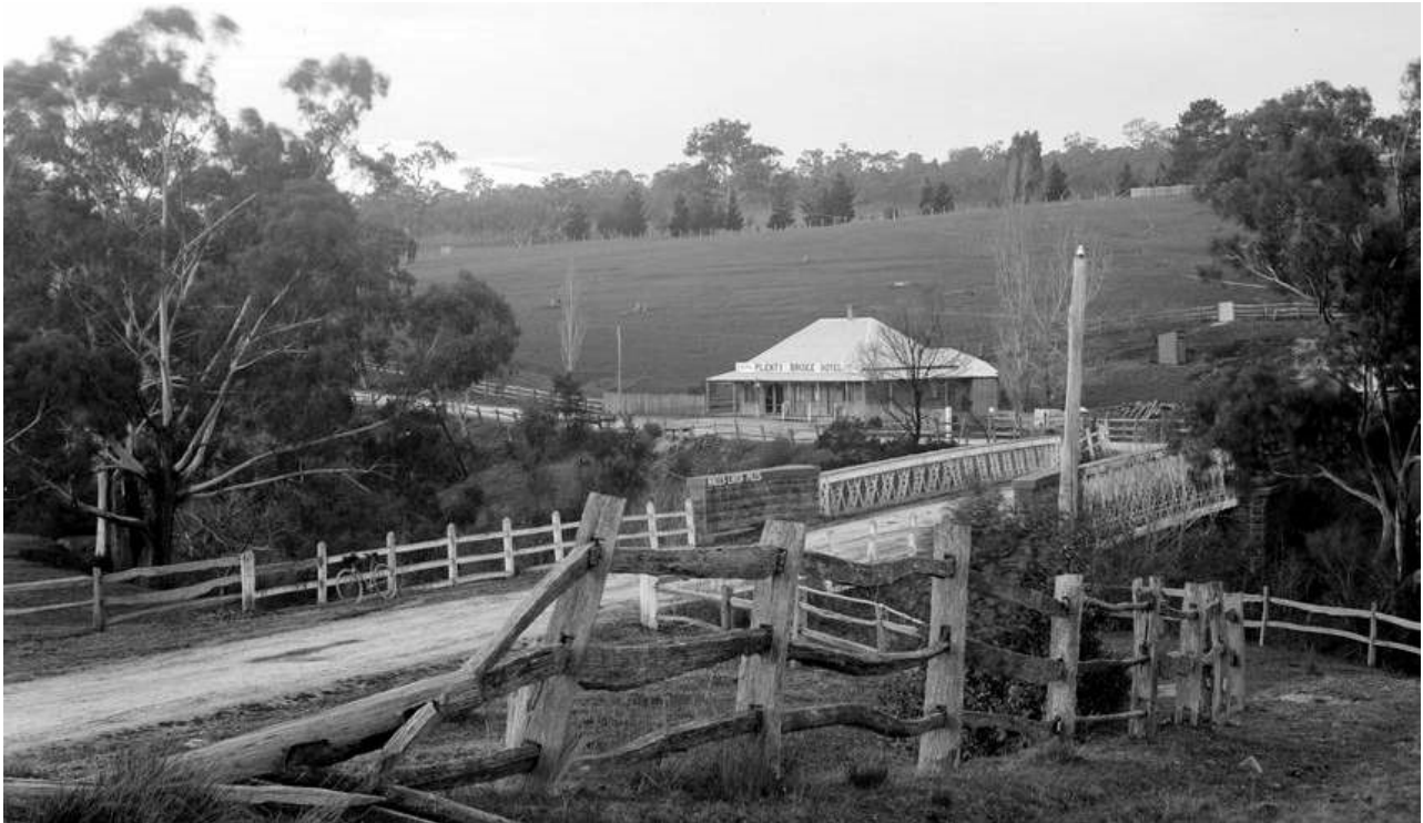
Figure 4.12 Plenty River bridge built in 1867. Photo c1900. Note the right angle bend created by creating the short length for the bridge.
