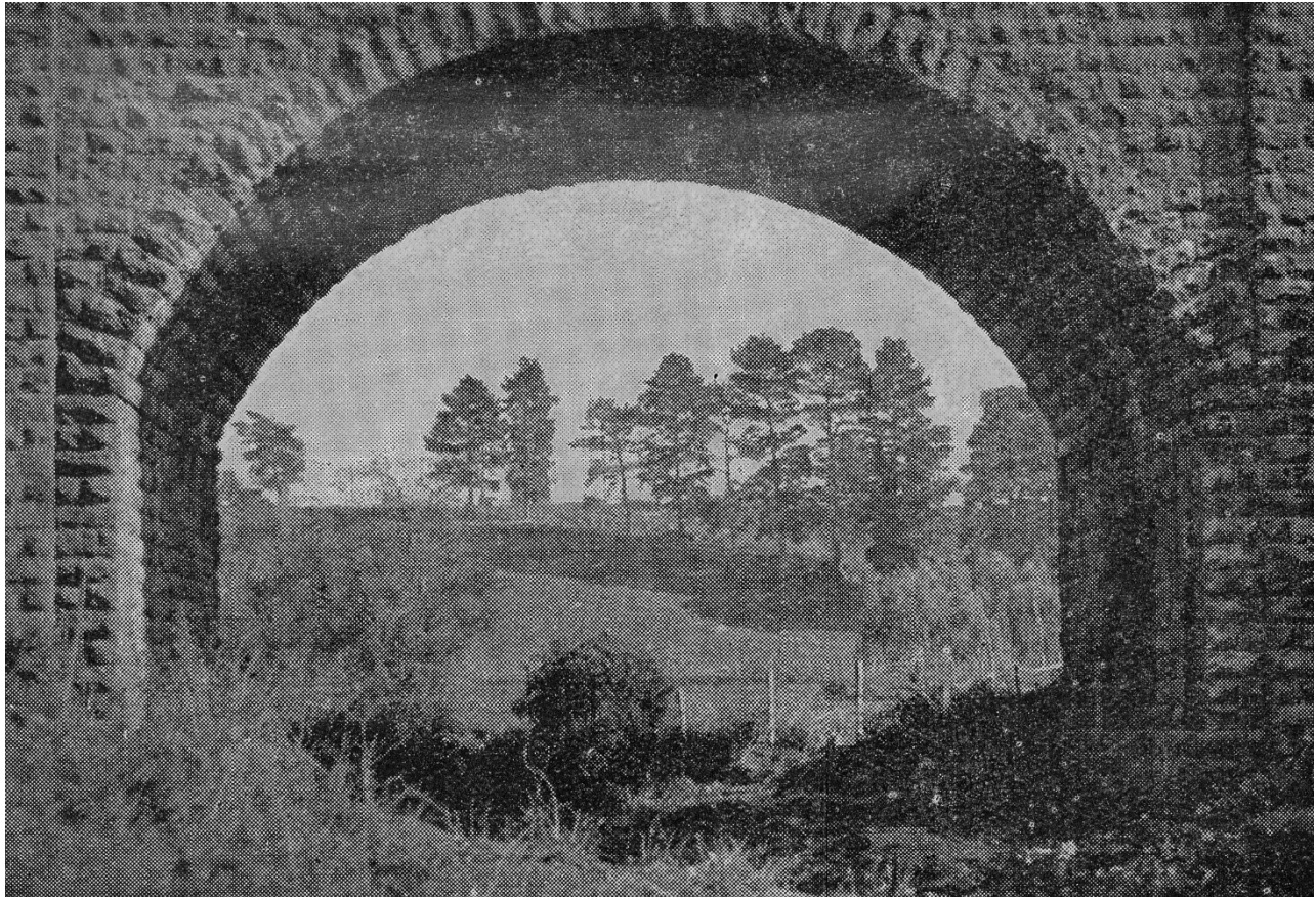
Figure 4.11 Heidelberg Rd bridge over the Darebin Creek, c1930
