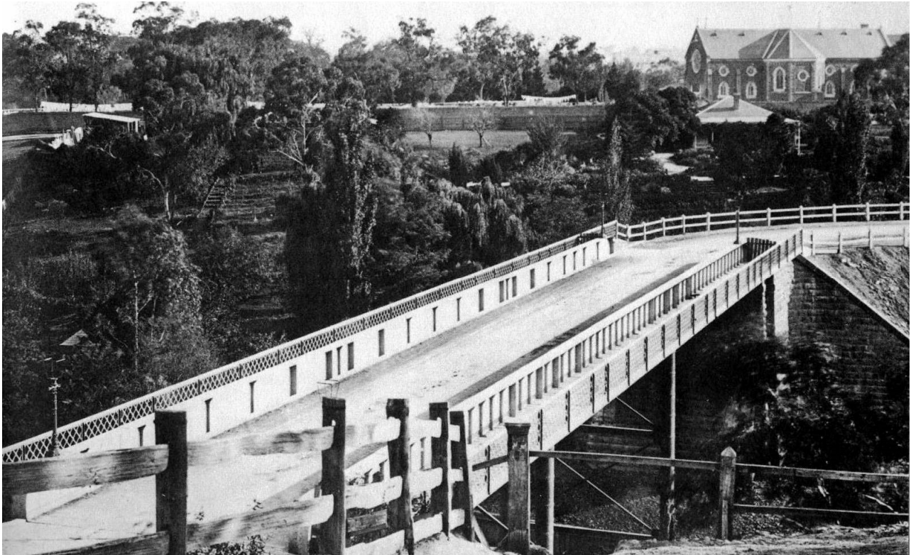
Figure 4.16 Third Johnstone St bridge, an iron girder bridge built in 1876 with three 18 m spans. National Trust
