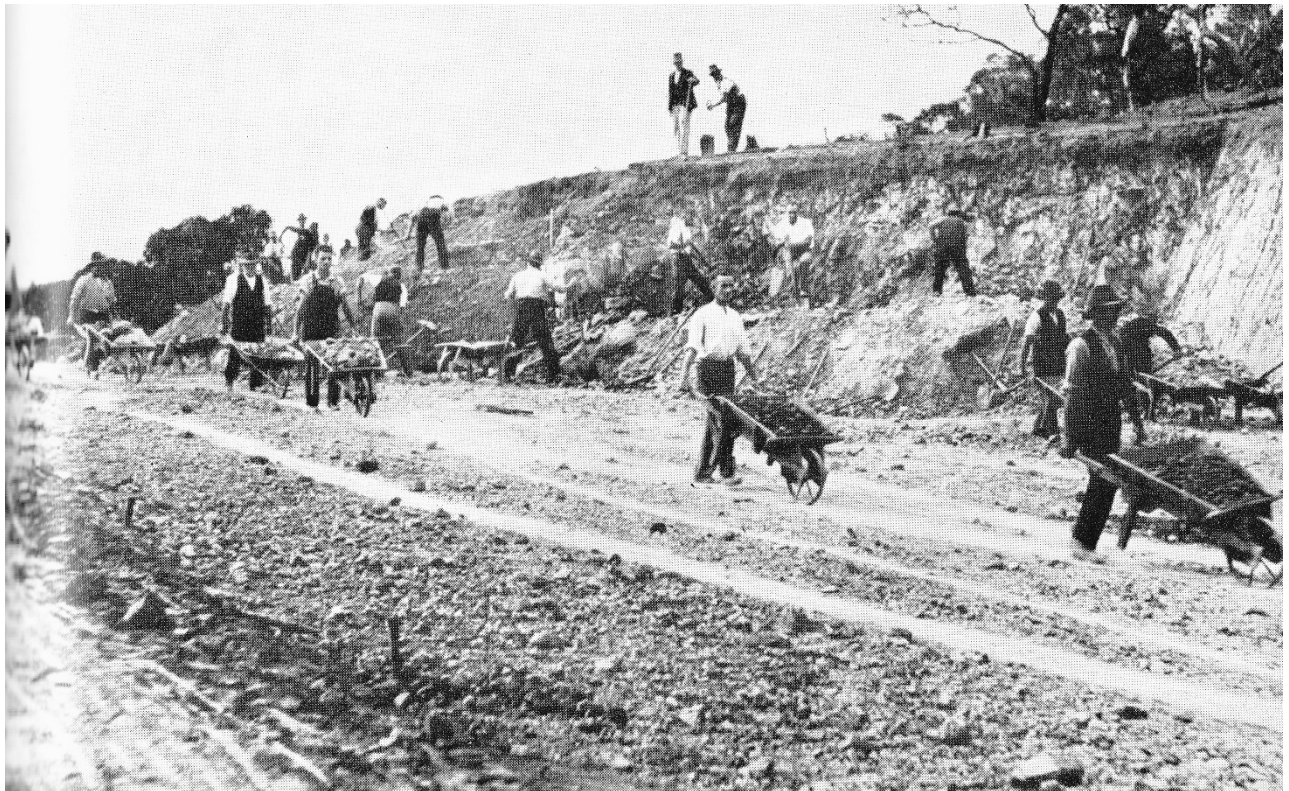
Figure 4.29 The Yarra Boulevard being hand-constructed by sustenance workers in 1934. Melbourne Herald
