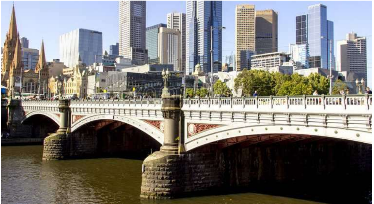
Figure 4.22 d’Ebro and Grainger’s 1888 Princes Bridge, looking upstream The Author
