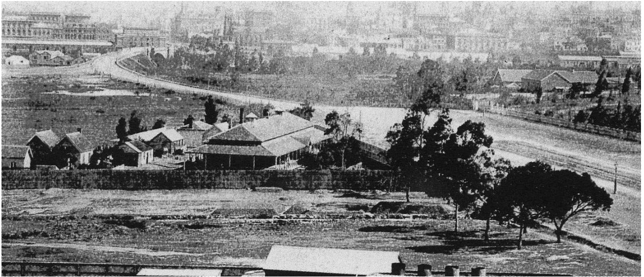
Figure 4.23 St Kilda Rd in 1865. Princes Bridge and City Rd are at top left and the Victoria Barracks is in the foreground. SLV
