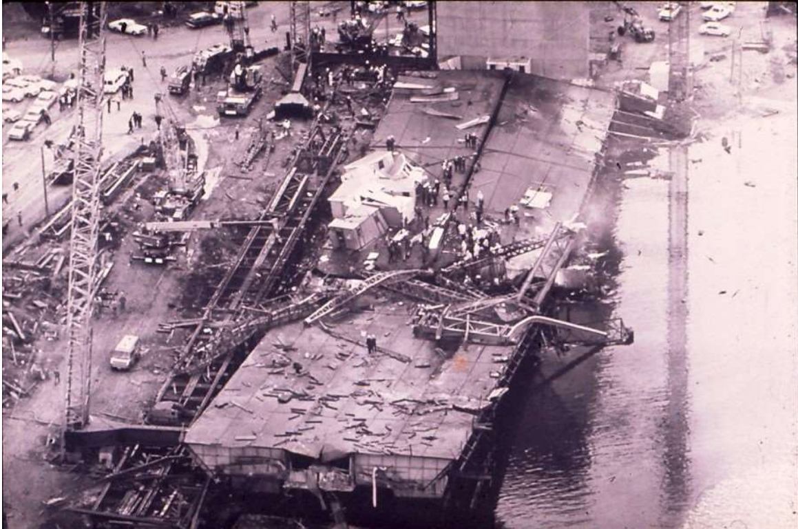
Figure 6.1 The collapsed Westgate Bridge in 1970. The span shown is across the Stony Creek estuary The Author
