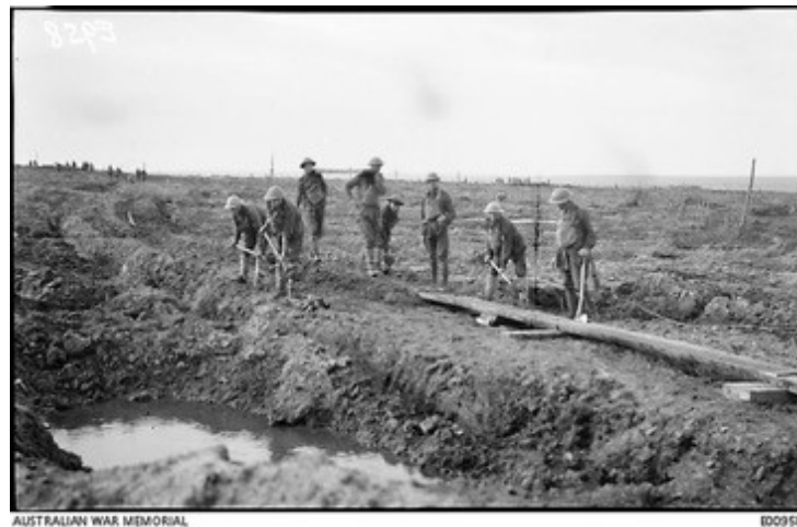
8th Field Company Sappers laying a mule track at Albania Wood near Ypres.
