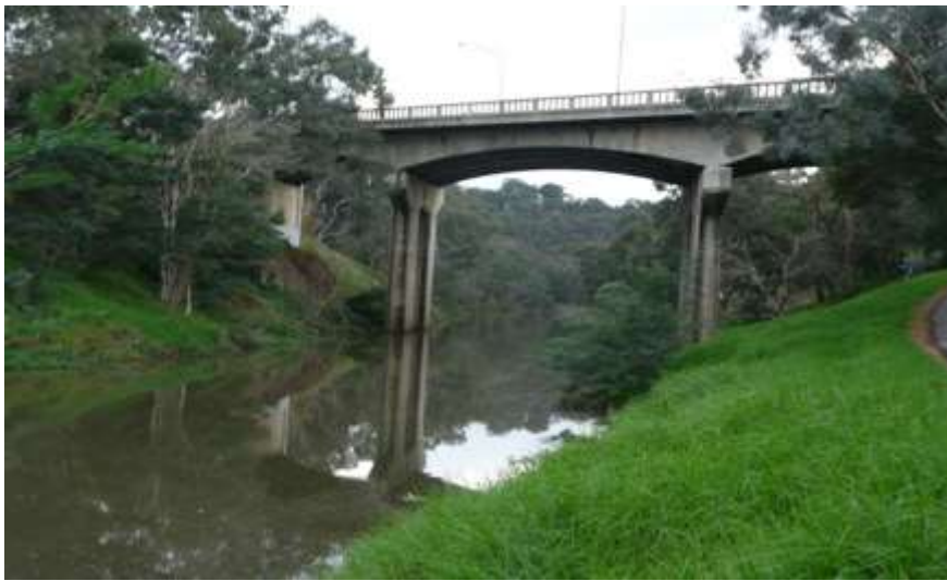
Johnston Street Bridge – Abbotsford.
