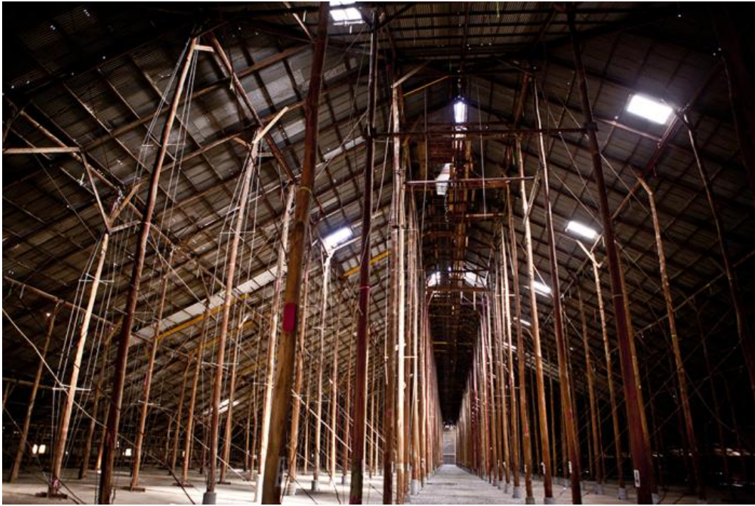
The Stick Shed at Murtoa.
