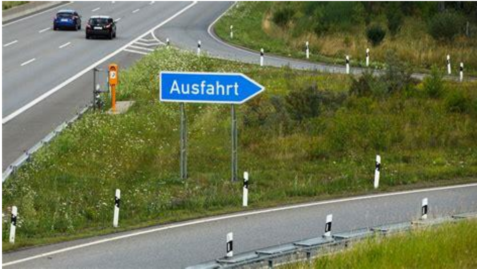
Low radius curves at the start/end of autobahn entry and exit lanes
