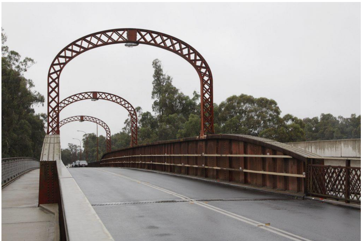
Looking north towards Moama along the original bridge - 2012.
