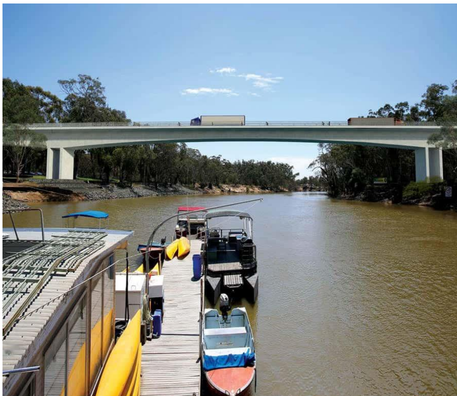
The new bridge at Echuca.
