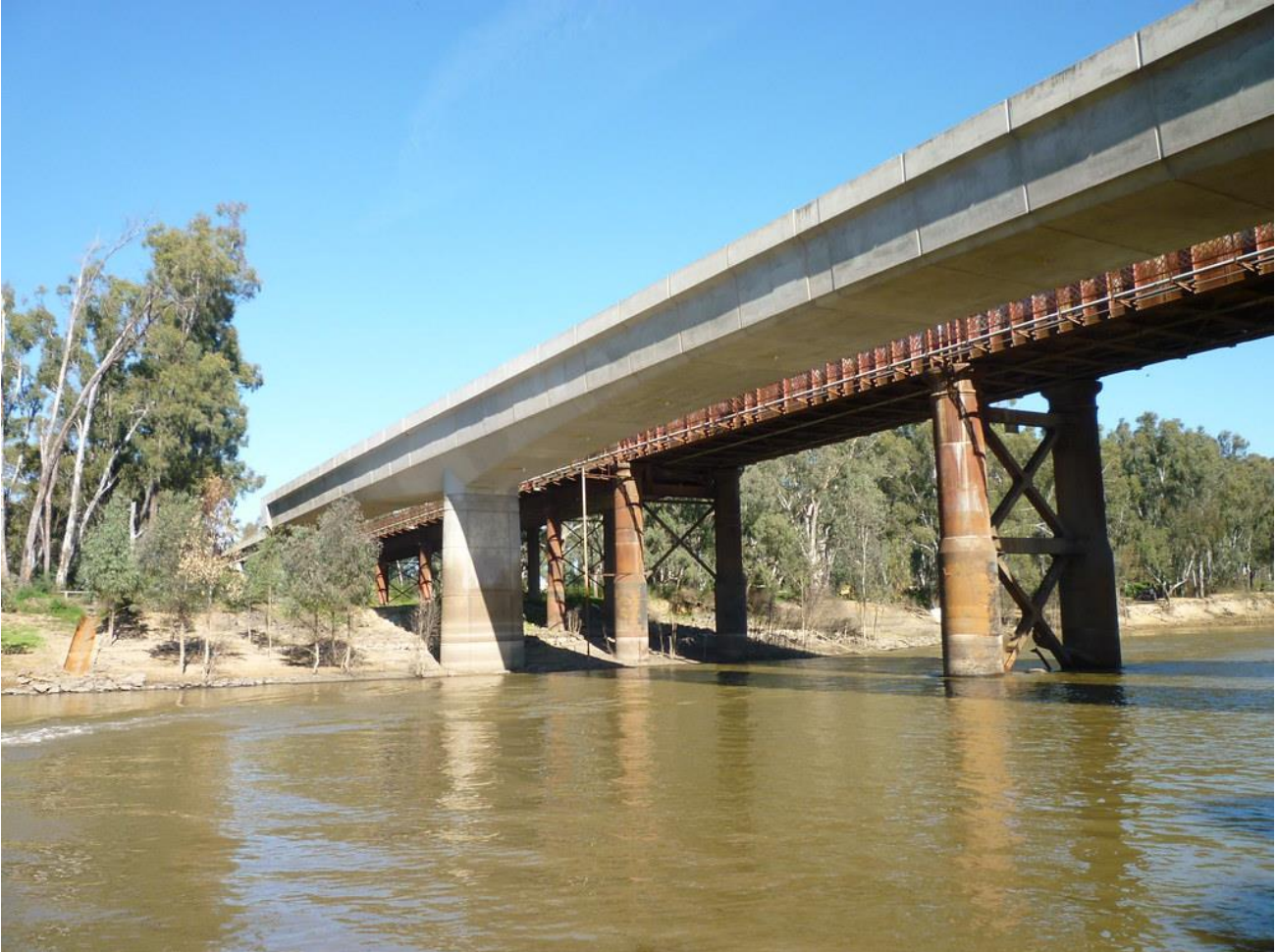
The new rail bridge beside the old road/rail bridge - looking downstream.
