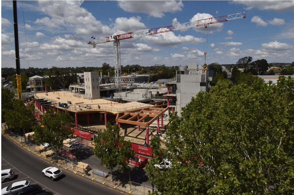
Galkangu under construction showing the timber framework.
