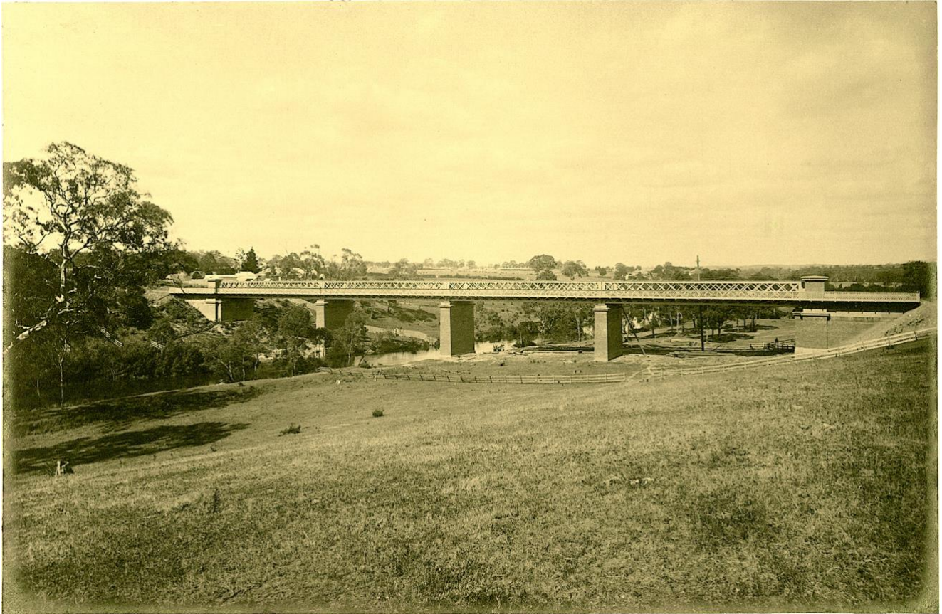
Chandler Highway Bridge – 1891.
