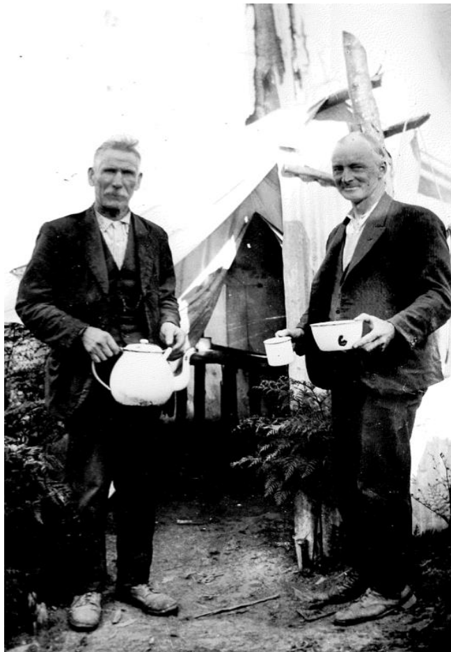
Mid 1930s – Men of the East Gippsland roads at 'home' near Bairnsdale
