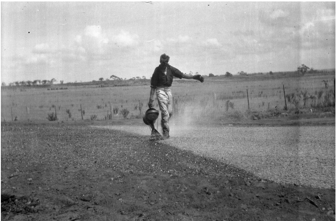
From 1938 – hand pouring seal on the Calder Highway
