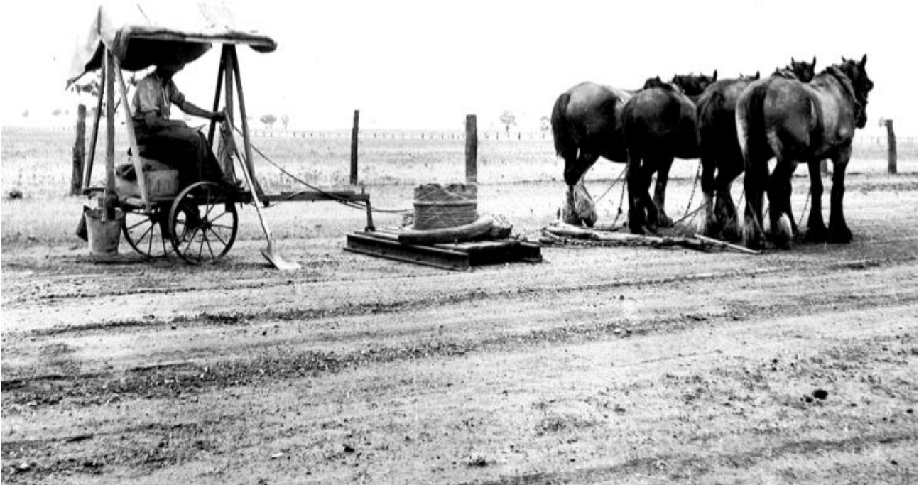
Circa 1936 – A patrolman's outfit for adverse weather conditions: dragging on the Serpentine Road in East Loddon Shire.
