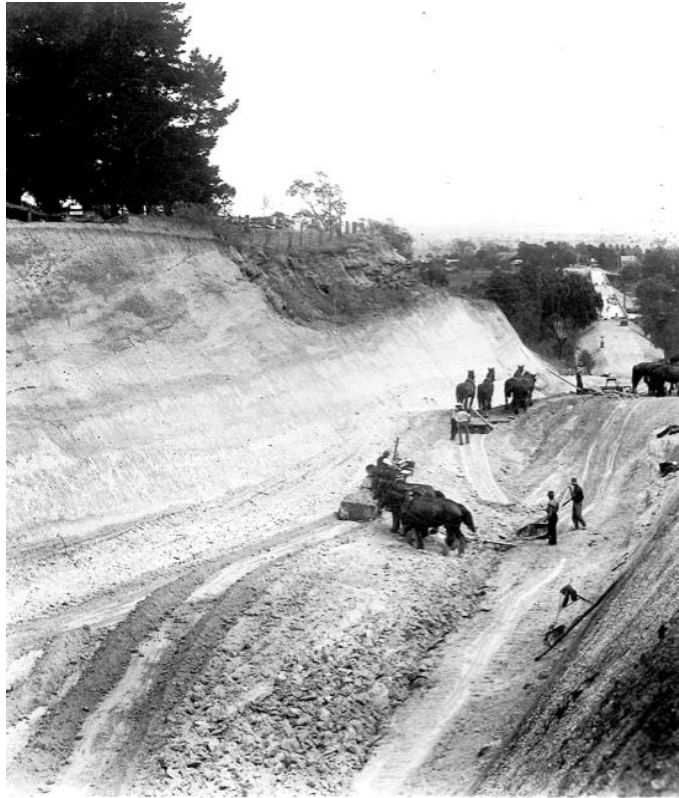
1937 – Building the cutting at Rosedale on the Princes Highway East – nearing the end of the horse era
