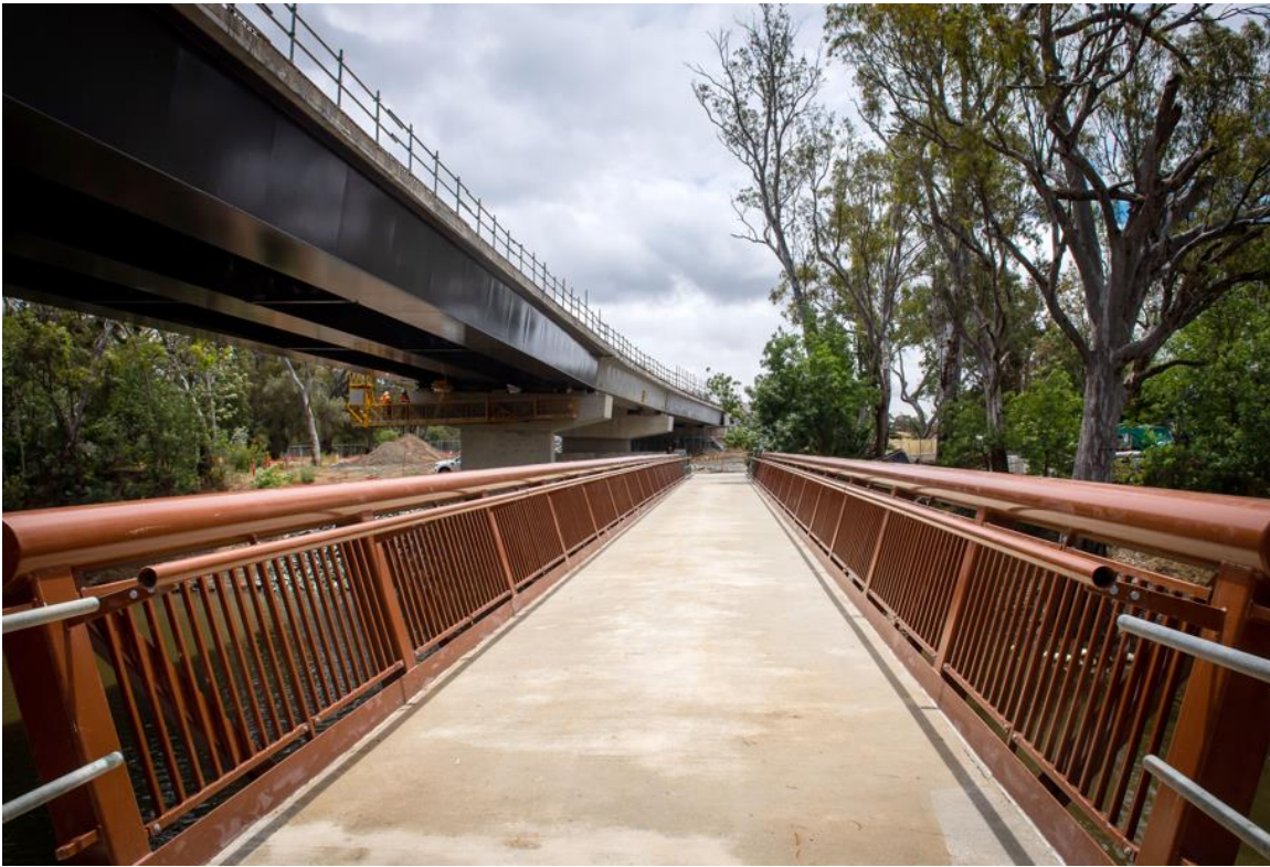
Pedestrian/cycle bridge across the Campaspe River – adjacent to the road bridge.
